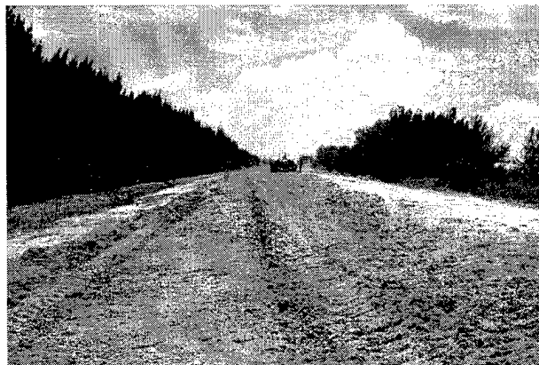
Figure 5. Incorporation of bagasse and N-Viro biosolids into sandy, droughty dredged material on Herbert Hoover Dike (Jun 95)
