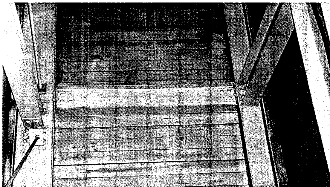
Figure A-2. Buckled horizontal brace (10-I-21), second floor between Columns P5.5 and N5.5.
