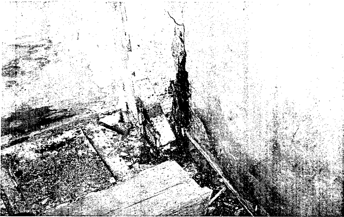
Figure A-5. Major corrosion sample retrieved from base of Column AO.5 (8-H-31).
