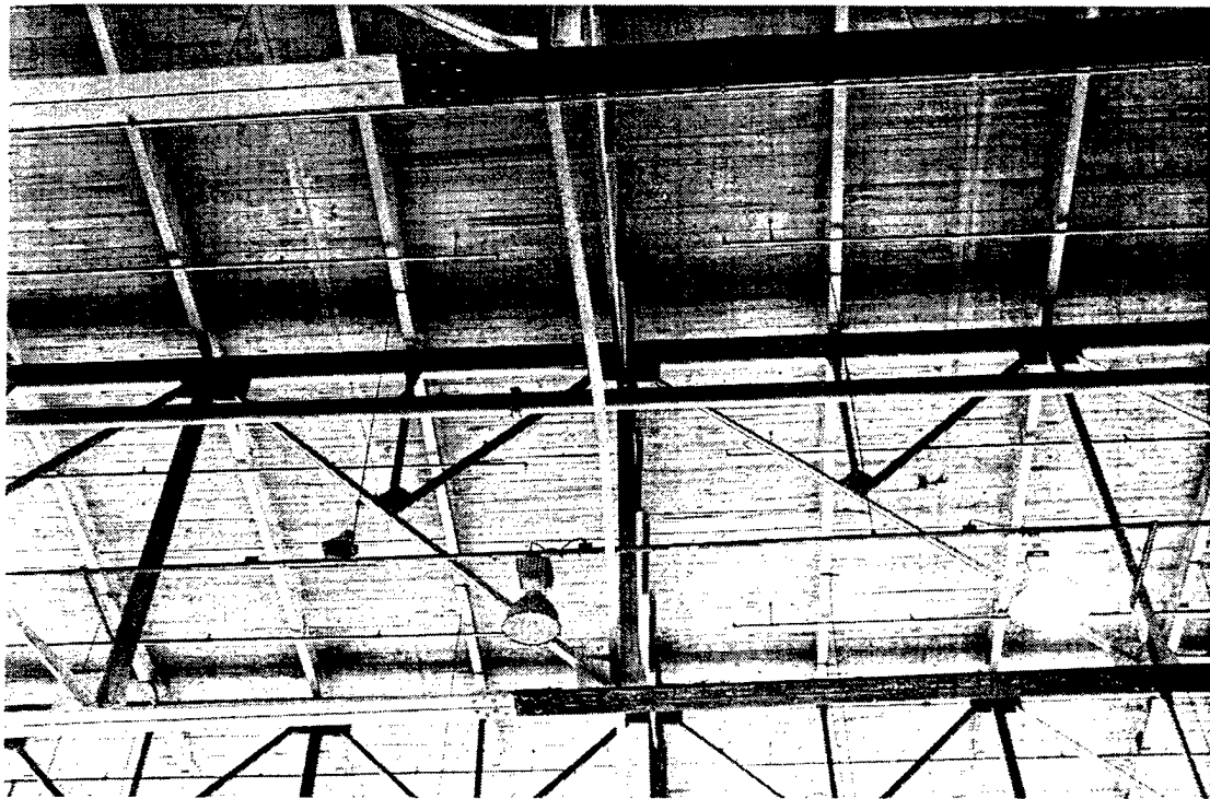
Figure A-18. Buckled bottom chord between Columns H3.2 and J3.2.
