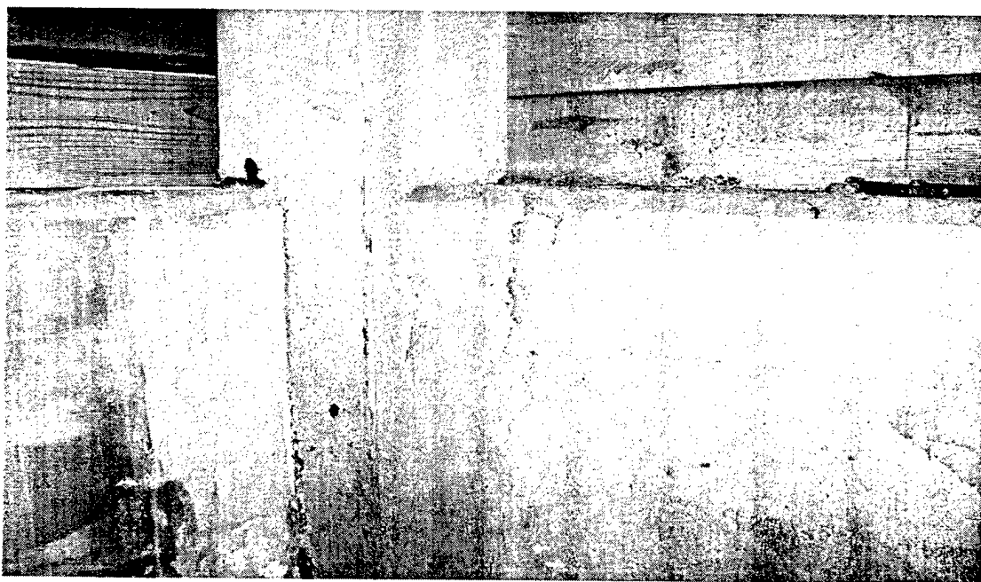
Figure A-4. Spalling concrete at the base of Column N5.5.
