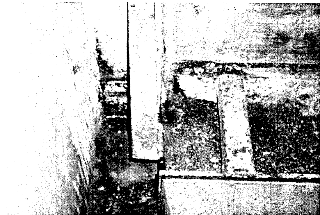
Figure A-9. Minor corrosion at the base of Column A5.5 (8-H-31).
