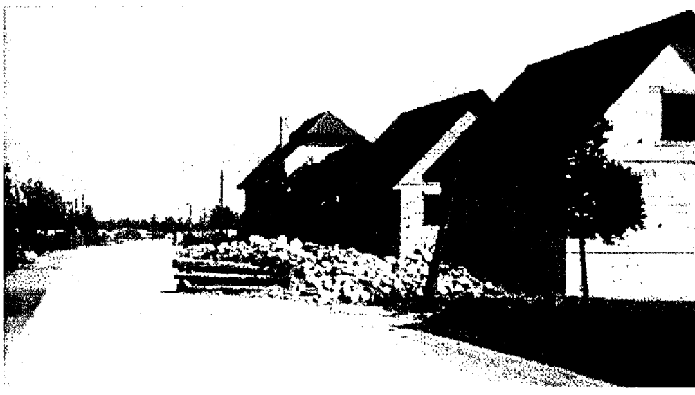
Figure 6.6—Photograph of Road at Copehill Down
