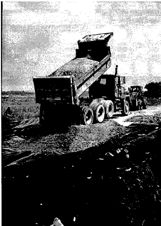
Figure 4. Placing fill soil inside the MESL.
