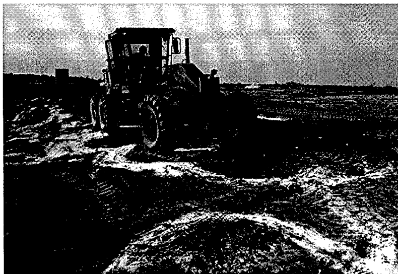
Figure 9. Grader mixing soil and lime.
