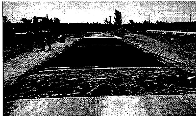
Figure 11. Completed puncture test section before placing a wearing surface.
