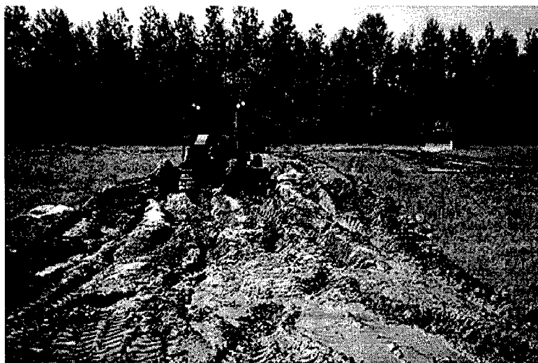
Figure 21. Mixing absorbent and soil together.
