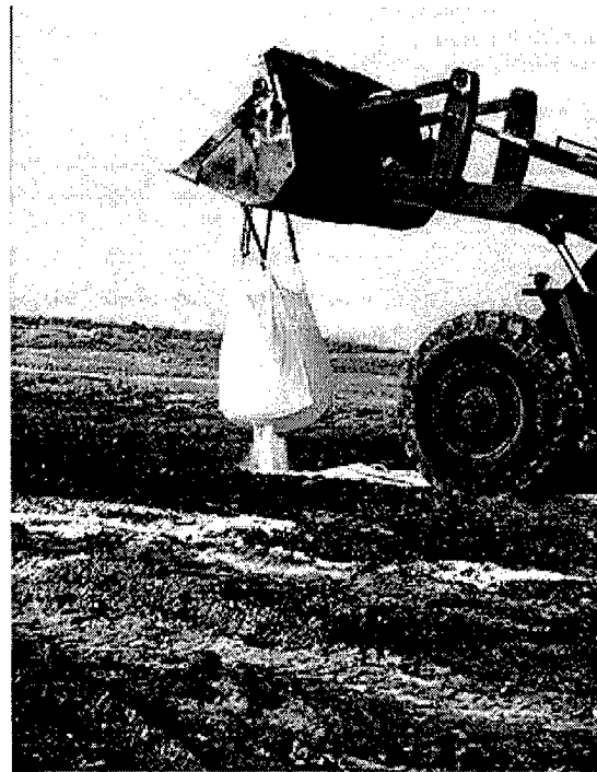
Figure 8. Bucket loader spreading lime.
