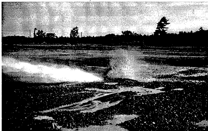
Figure 16. Washing gravel.
