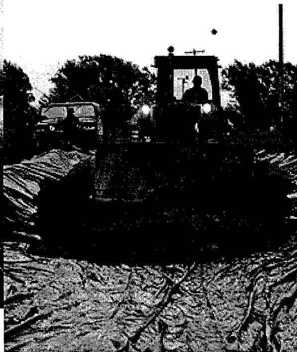
Figure 5. Using a D-7 to spread soil in the MESL.
