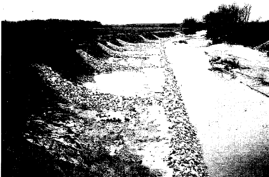
Figure C5. Longitudinal stone fill toe protection riverward of high bank with tie backs
