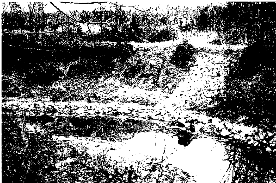
Figure C2b. Typical longitudinal peaked stone toe protection with tiebacks
