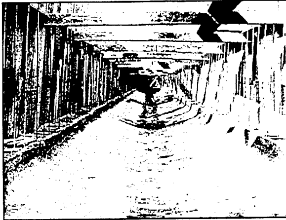
Figure 69. Interior of the Hagan Avenue Canal, shown during construction, ca. 1906. This concrete-lined and covered canal was constructed 1904-1906 (from Sewerage & Water Board 1906a).
