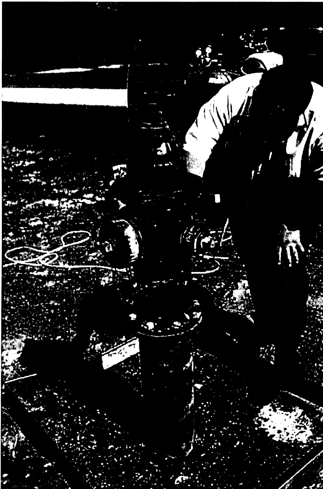
Figure F- 7. Wire brush cleanup of hydrant near Building 6029 after TSV application.
