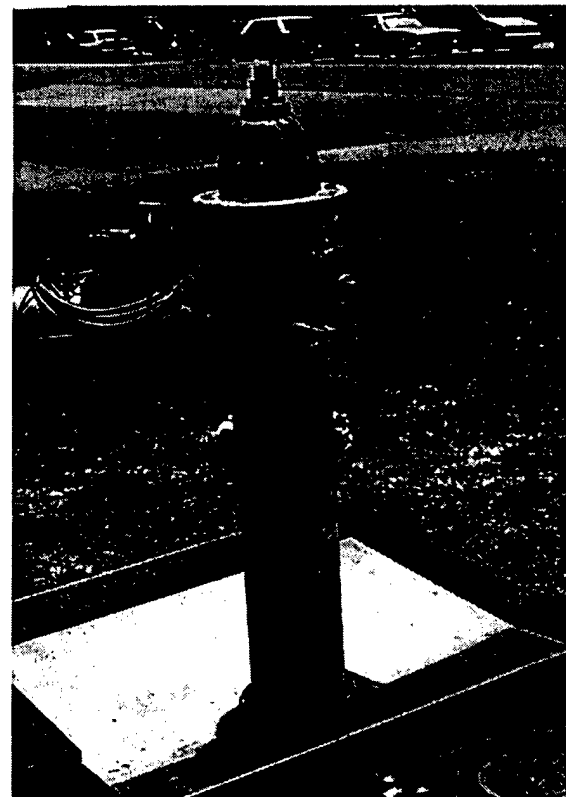
Figure F- 4. Fire hydrant near Building 6029 with collection pan.
