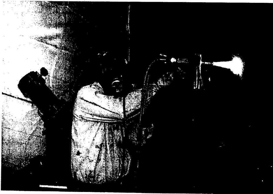
Figure B-2. Application of TSV process to Viaduct Bridge at the Rock Island Arsenal.
