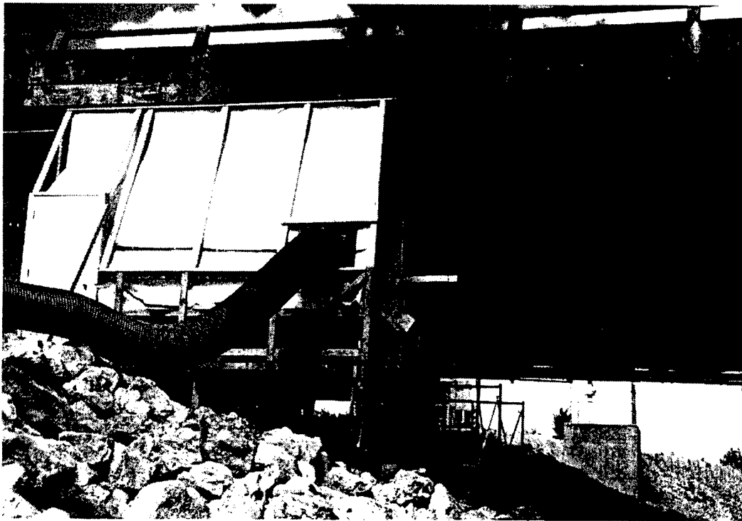
Figure B- 6. Containment structure built for the Rock Island Bridge demonstration.
