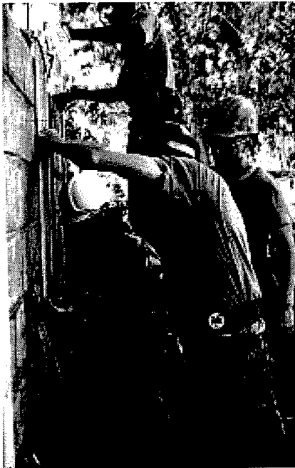
U.S. Army Pacific and Royal Thai Army engineers work side-by-side to construct a schoolroom during COBRA GOLD '97 in Thailand.
