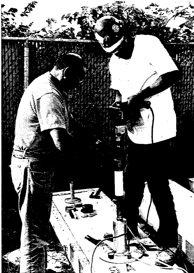
Figure 9. Core drilling
