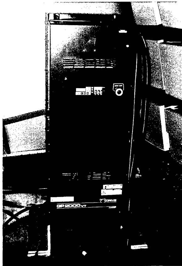
Figure 16. Test Article: Reliance Electric Motor Controller.
