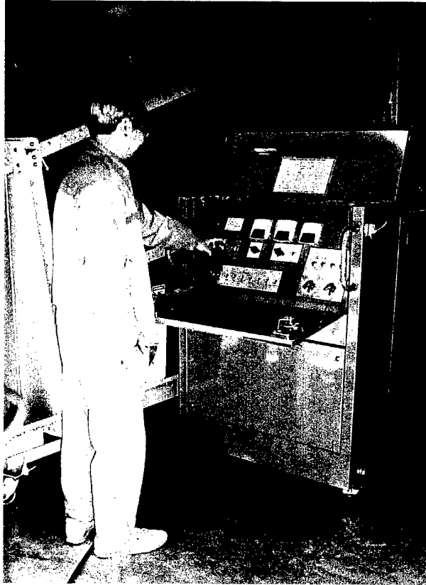
Figure 8. Resistive load bank.
