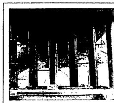
A view of columns repaired and strengthened with carbon and glass fibres, ready for painting
