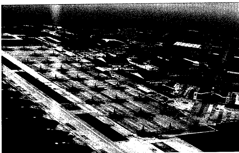
Military air bases with the capacity for supporting increased workloads are demobilized during peacetime, but can be activated to provide the needed facilities for conducting airlift staging operations during mobilization.
