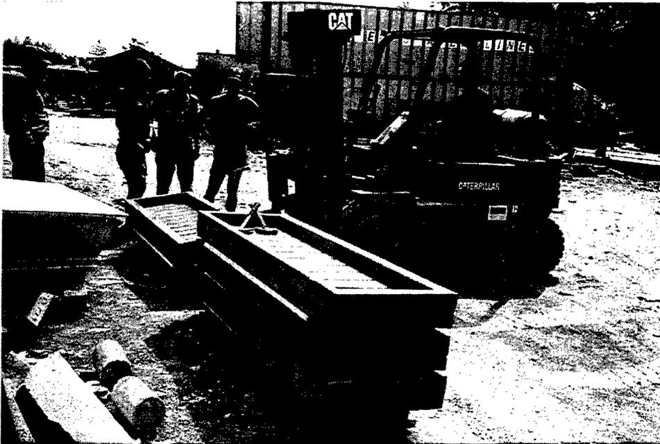
Figure 5. Preparing precast concrete test slabs for shipment
