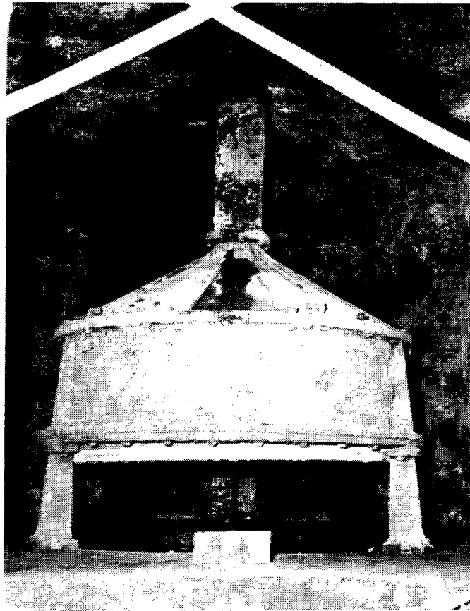
Figure 22. Photograph of "cylindrical drum type gate" or valve taken during 1970 dewatering. (Courtesy NOD)
