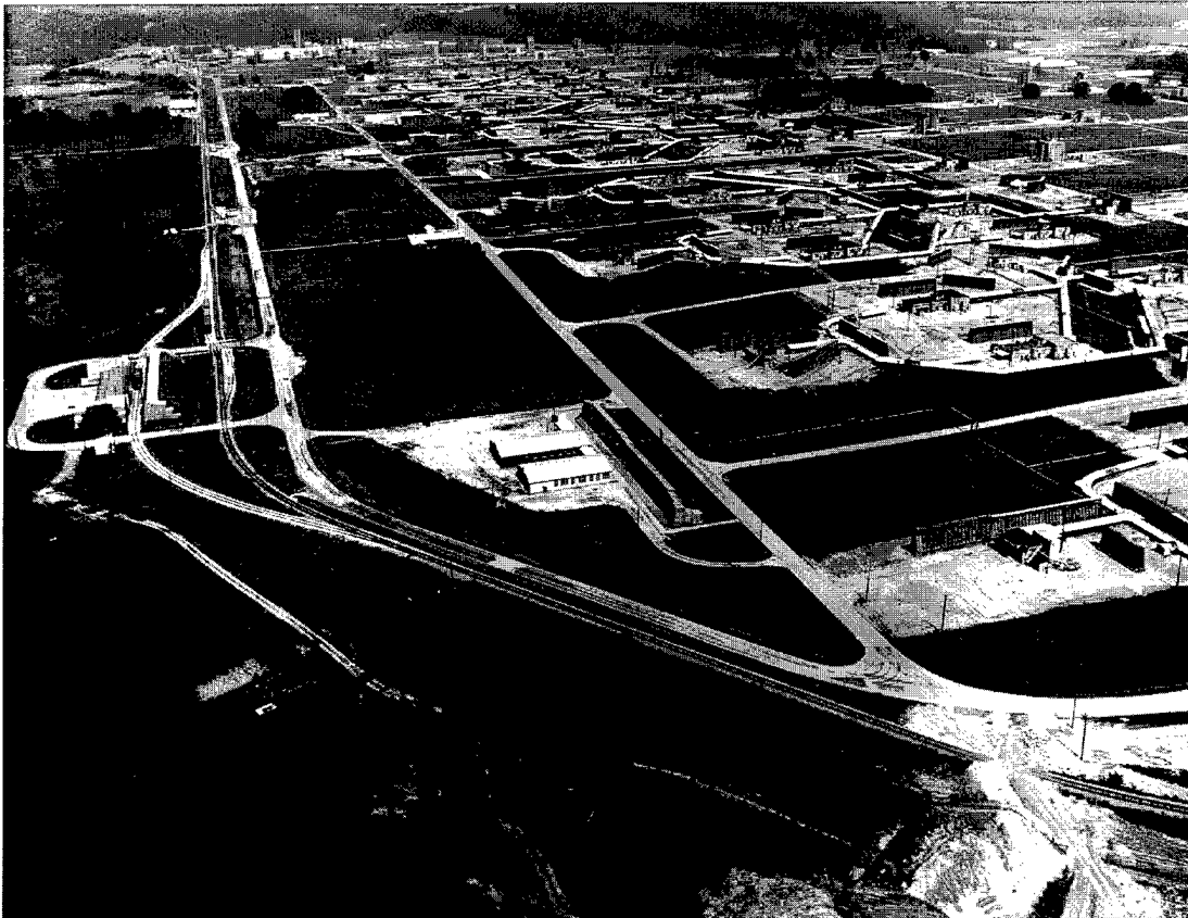
Production lines for the manufacture of the high explosives RDX and Composition B at Plant B, Holston Army Ammunition Plant. Note the covered walkways and the blast barriers that isolate and shield each of the manufacturing buildings on the enormous plant complex. Source: Holston Army Ammunition Plant.
