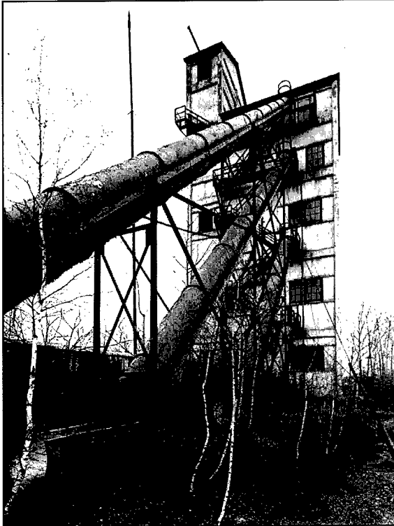
Building 561, Cannon Powder Blender, Picatinny Arsenal. Note the escape chutes to allow the workers to escape the building quickly. Source: HAER No. NJ-36C-83, Picatinny Arsenal, Prints and Photographs Division, Library of Congress.
