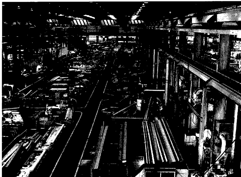
The Shipfitters Shop at Puget Sound Naval Shipyard, January 1963. This shop is where the parts of the ship's hull were laid out and assembled during construction. Source: Puget Sound NSY, Photo No. YV-832.
