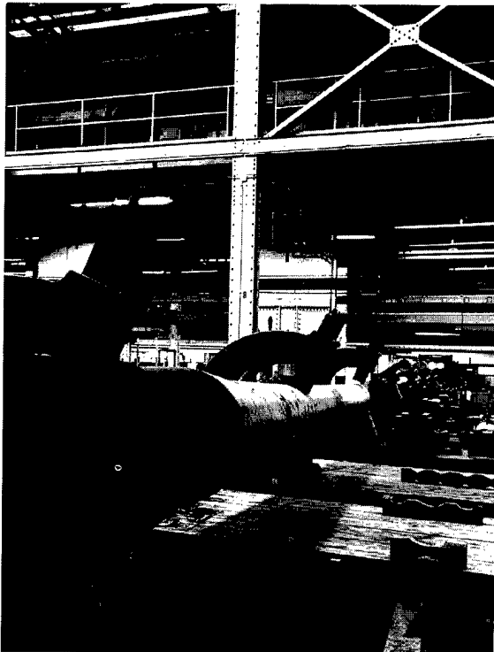
Sixteen-inch gun tube mounted on machining lathe, Big Gun Shop (Building 110), Seacoast Gun Shop, Watervliet Arsenal. The gun extends beyond the main bay of the shop and into the West Aisle. Source: HAER NY-1B-62, Watervliet Arsenal, NY, Prints and Photographs Division, Library of Congress.
