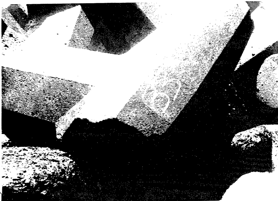
Figure 19. Dolos with straight fluke-shank break
