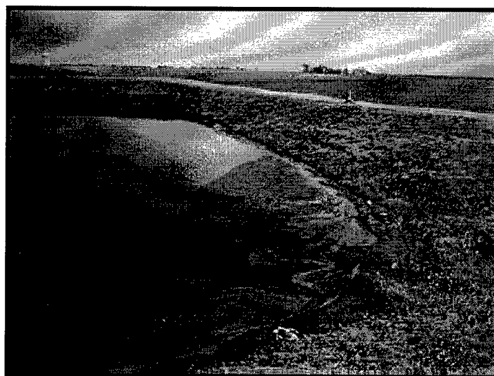
Figure 4. Kirkwood Community College two-stage anaerobic hog manure lagoon (1st stage).
