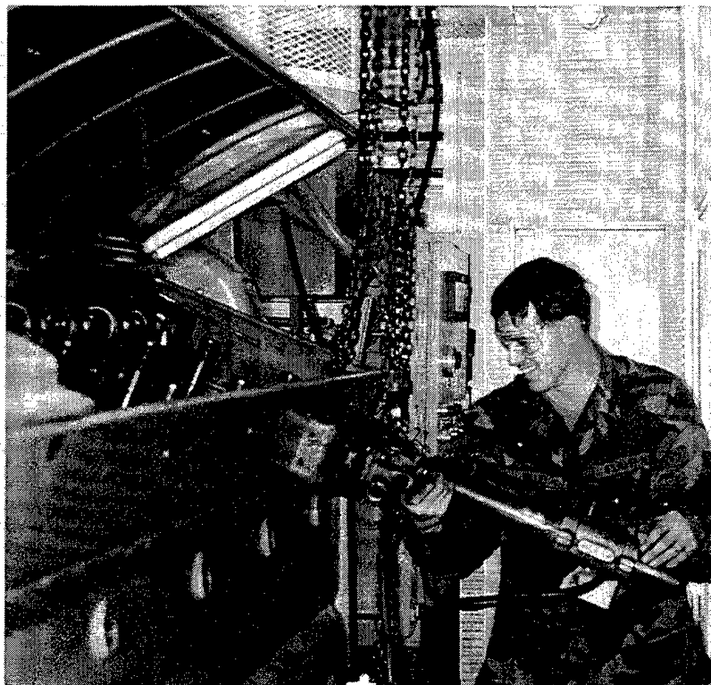
(i) Installing an NG load block.
