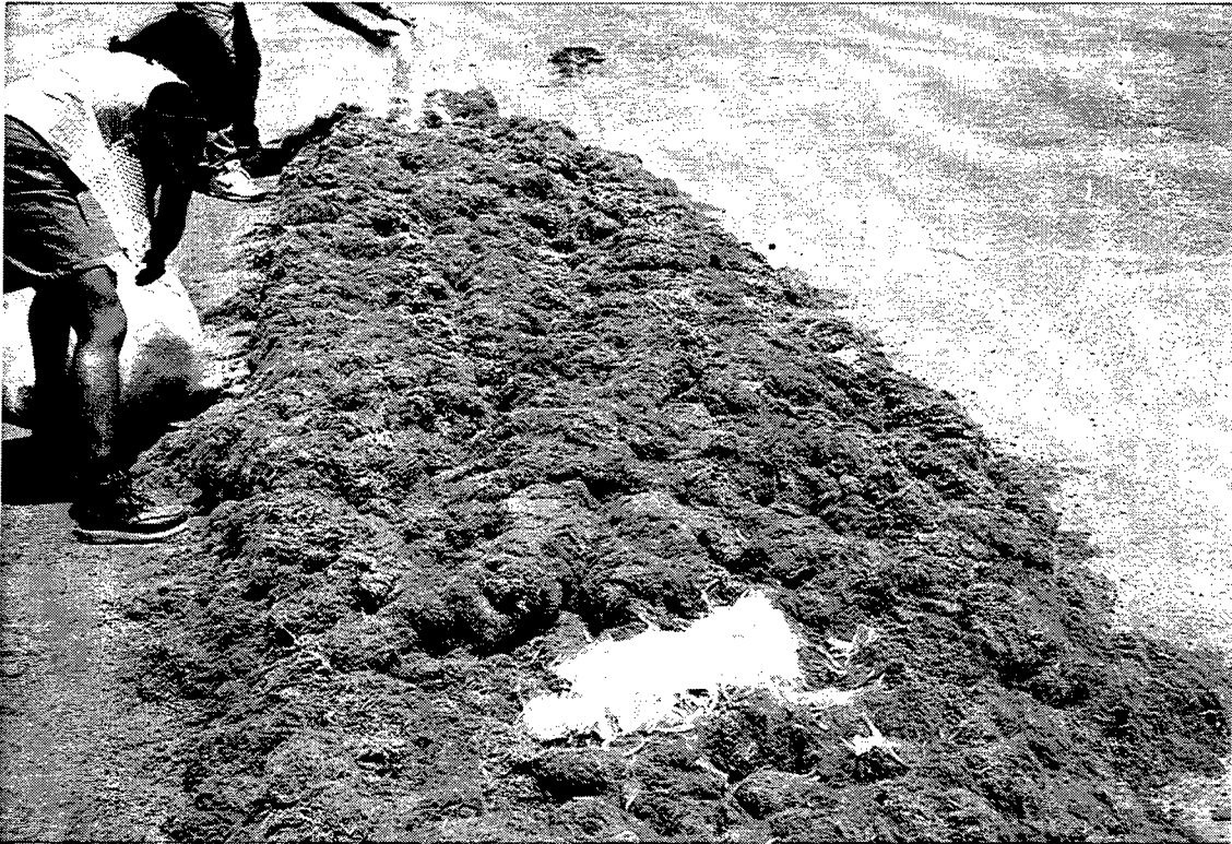
Figure 5. Fiber mixed in sand after four passes
