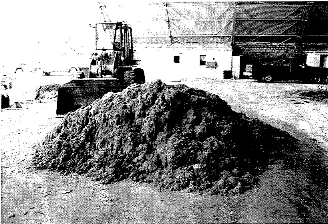
Figure 35. Mixture of sand-fiber and Road Oyl prior to installation
