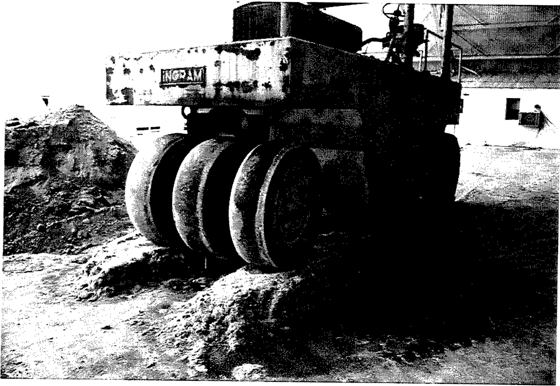
Figure 7. Sand-fiber ramps with 50,000-lb compactor
