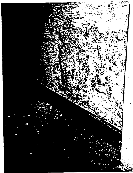
Figure 27. Wall leaks can cause historic surfaces to deteriorate, thereby exposing underlayers of lead-based paint. If painted surfaces show signs of deterioration, they should be repaired as soon as possible.
