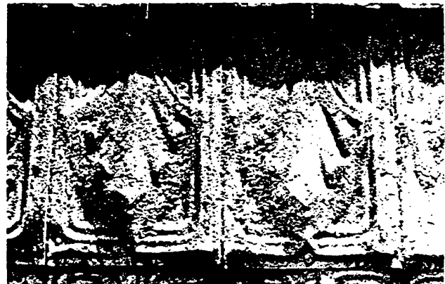
Tin shingles, commonly embossed to imitate wood or tile, or with a decorative design, were popular as an inexpensive, textured roofing material. These shingles 8 3 / 8 inch by 12 1 / 2 inch on the exposed surface were designed with interlocking edges, but they have been repaired by surface nailing, which may cause future leakage. (Ballard House, Yorktown, Virginia, photo by Gordie Whittington, National Park Service)
