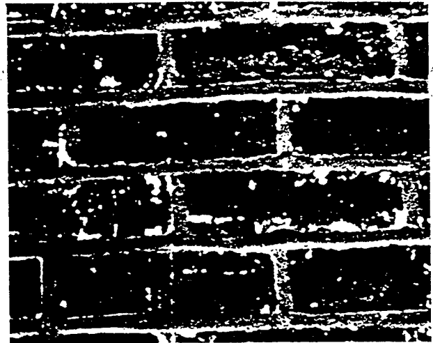
Abrading the Surface without Removing the Paint. Even though the entire outer surface layer of the brick has been sandblasted off, spots of paint still cling to the masonry. Sandblasting or other similarly abrasive methods are not always a successful means of removing paint.
