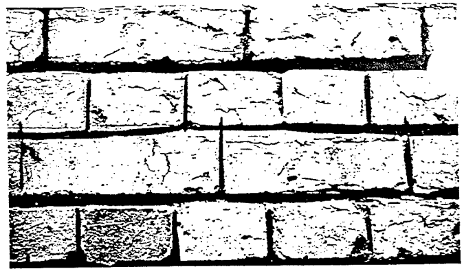
Figure 5. The damage to these bricks was caused by using a power saw with a carbide blade to rake out the mortar joints. Note the overcutting of the joint into the brick above the vertical joint. Careful hand work is required to prevent such damage to the brick during joint preparation. Photo: John Myers.
