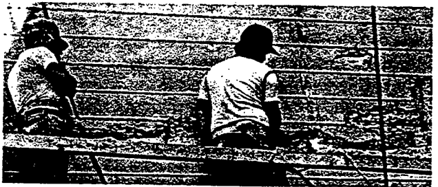
Fig. 13d. Deteriorated or redundant reinforcing bars are removed after evaluation by a structural engineer. An acetylene torch is being used to cut out the bars.
