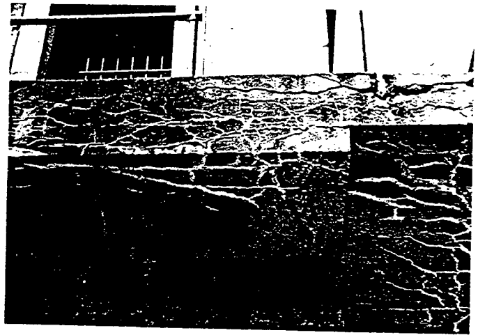
Fig. 7. Battery Commander's Station, Ft. Washington, Maryland (1904). This reinforced concrete tower with a cantilevered balcony is showing serious deterioration. Water has penetrated the slab, causing freeze-thaw spalling around the posts and corrosion of the reinforcing bars. This internal corrosion is causing expansion inside the slab and creating major horizontal cracks in the concrete. Under the balcony can be seen the network of hardened white calcified deposits, which have exuded through cracks in the concrete as a result of alkali-aggregate reaction. Photo: Lee H. Nelson, FAIA.
