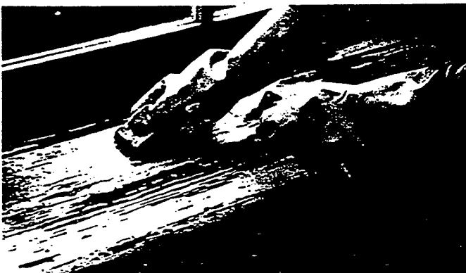
Figure 15. Wet sanding of interior surfaces will keep dust levels down, reduce the need for workers' protection, and provide a sound surface for repainting. Priming and repainting with oil/alkyd, latex or latex acrylic should be undertaken according to manufacturers' instructions.
