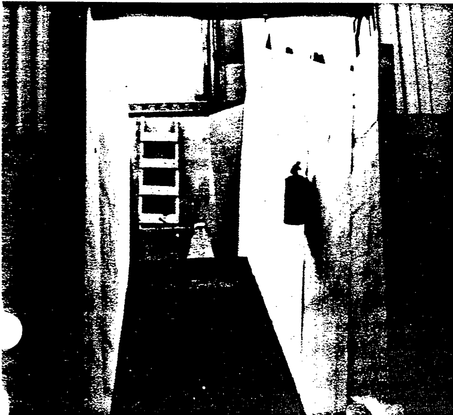
Figure 8. The entire historic staircase has been protected against possible damage during the renovation work. The balustrade on the left has been encased in plywood; the floors have been covered; and a temporary plywood wall constructed, shown on the right and at the landing. Note that the plywood wraps around the wall at the entranceway. Photo: Charles Fisher.
