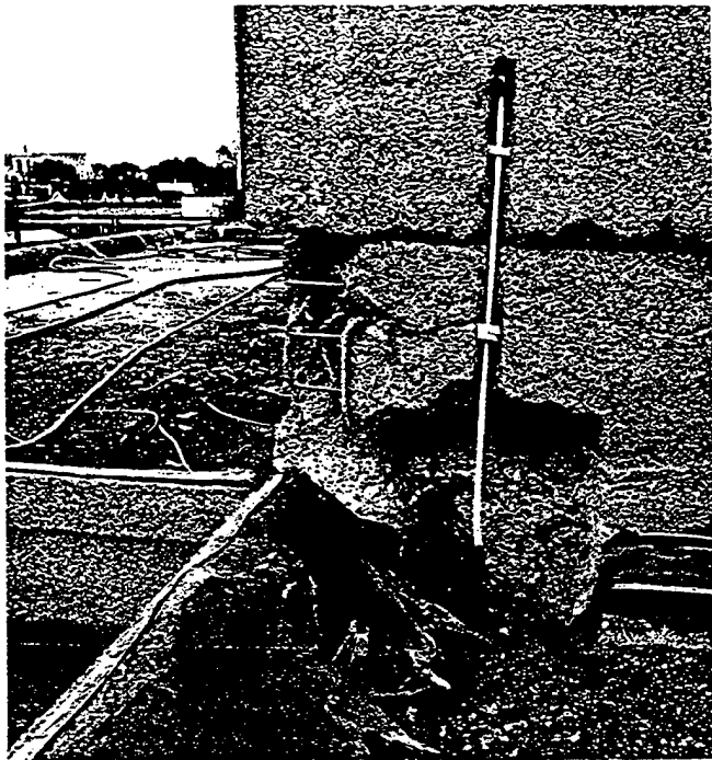
Fig. 14a. Spalled concrete was most noticeable at locations of concentrated rebars. Deteriorated concrete, the 1960s stucco finish, and corrosion were removed by grit-blasting. Photo: Robert Bell.
