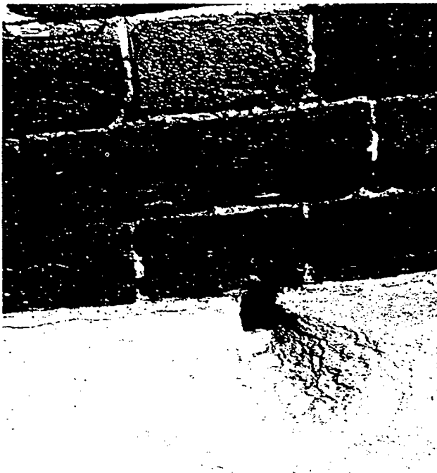
Figure 1. The iron anchor shown here originally was hidden from view. An increase in volume due to rusting created internal pressures on the stone and brick, causing spalling. Careful study of the building construction can result in the identification of these potential problem areas and they can be taken into consideration while planning a cleaning project.
