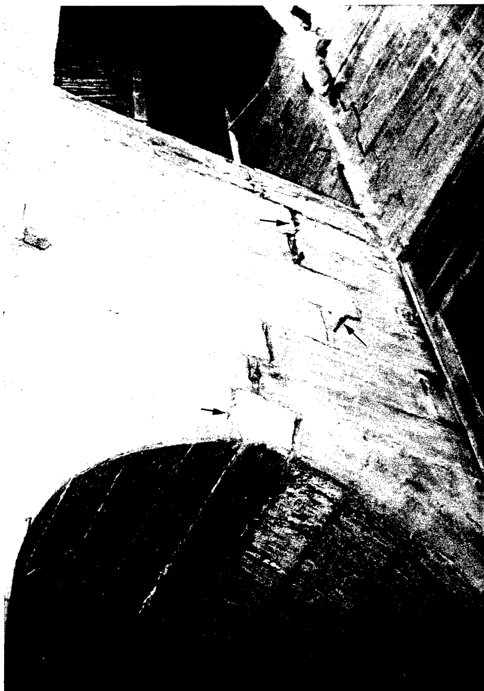
FIGURE 4-13 Wall at southern corner of inner court of Mosque of Sultān Barqūq showing crack in southwestern wall extending down to arch
