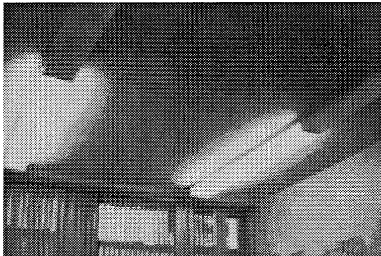
Figure 7.6. The Back Lights in the Classroom are Turned on Separately and All Four Banks are Now Independent.
