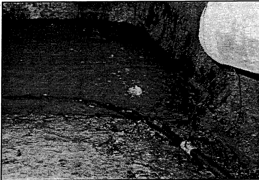
Figure D-28 Gas (Methane) Seepage at Sta. 18+50
