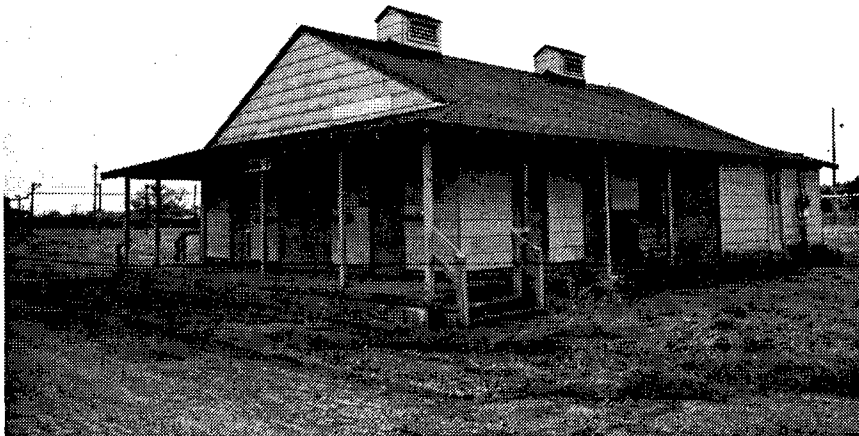
Figure 163. Building 6816-1: Final Inspection House.
