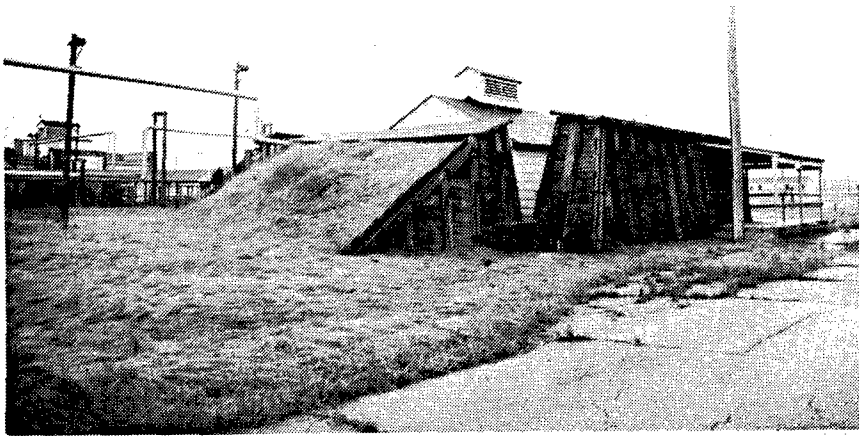
Figure 309. Building 6882-1: Final Rest House. Completed ammunition products waited in such structures until they could be transferred to a Magazine for more permanent storage.
