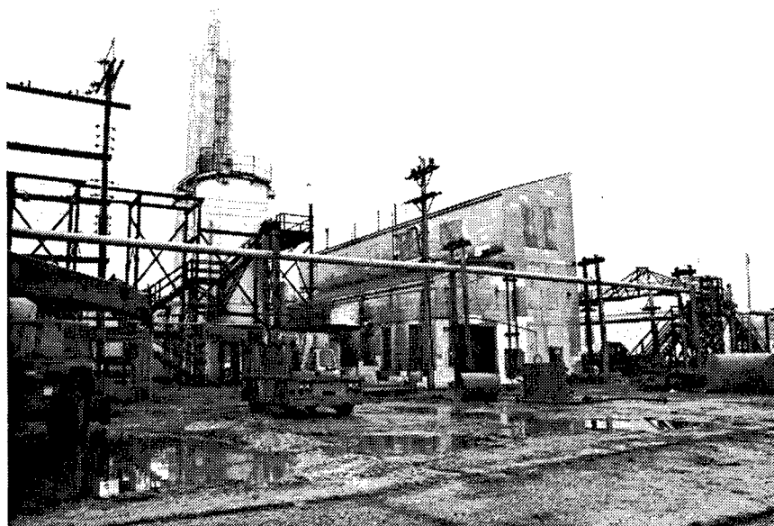
Figure 38. Building 728: Oleum Manufacturing Plant. The oleum produced here was used in the nitrating of cellulose.
