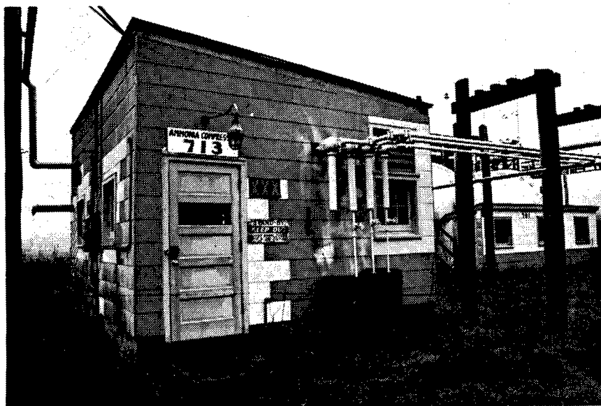
Figure 36. Building 713: Ammonia Compressor House.
