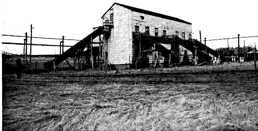
Figure 116. Building 6701: Nitrocellulose Blender House.
