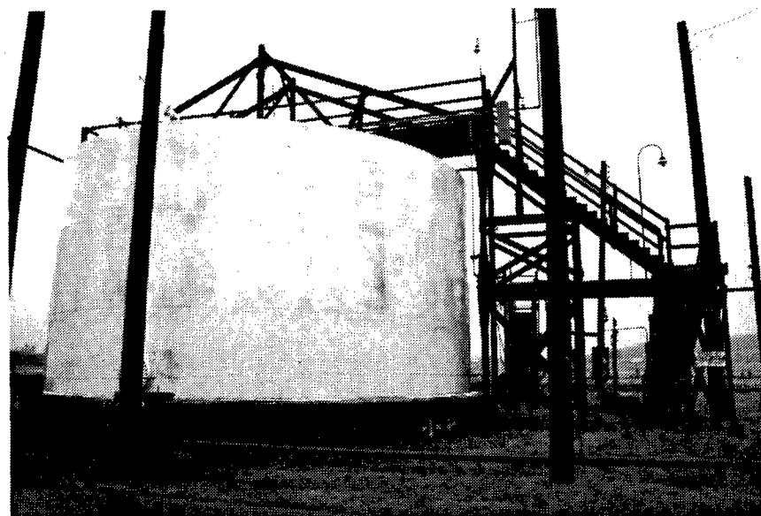
Figure 29. Building 704-1: Storage product tank for 92% sulfuric acid.
