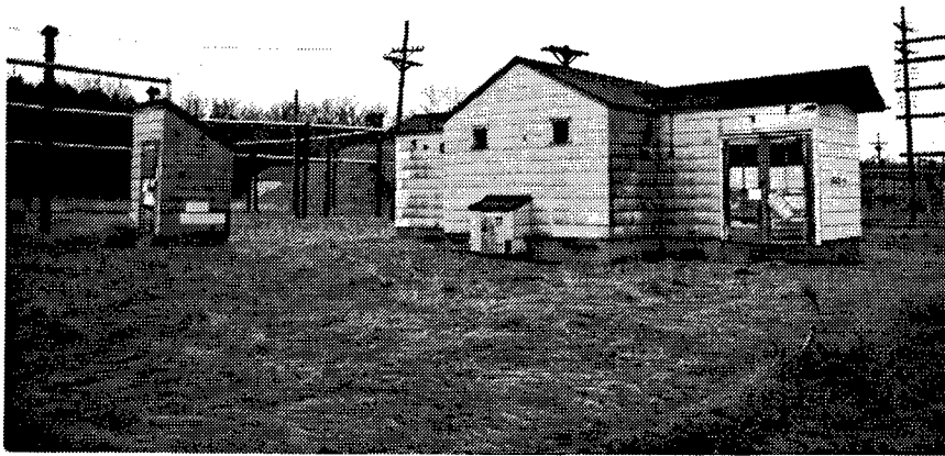
Figure 158. Building 6812-11: Rest and Heating House, not barricaded.
