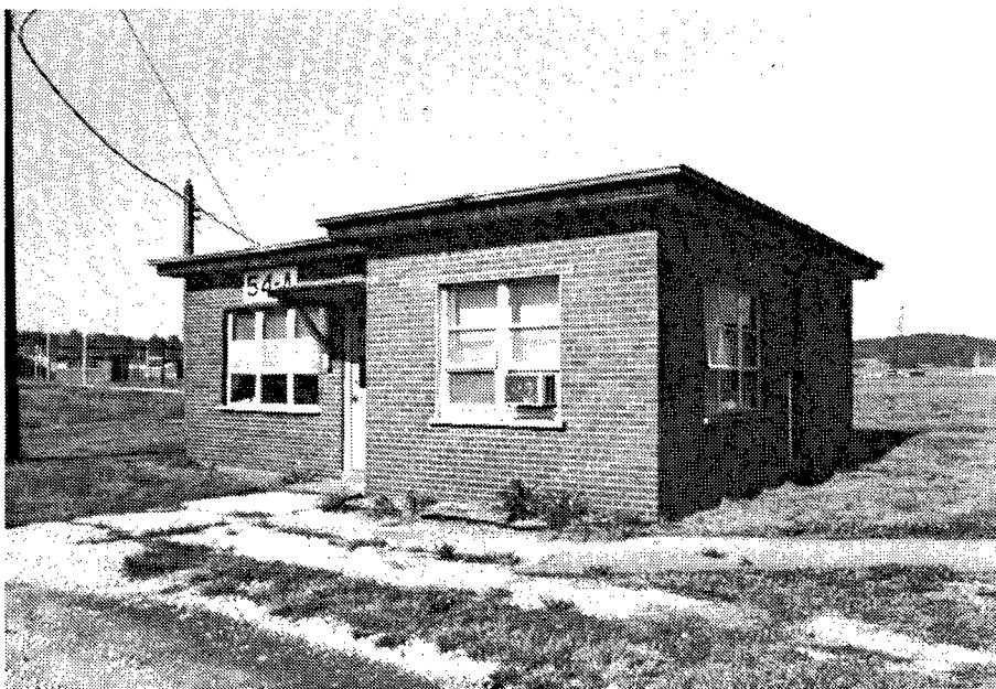
Figure 228. Building 54A: Change House and Attendant's Station.
