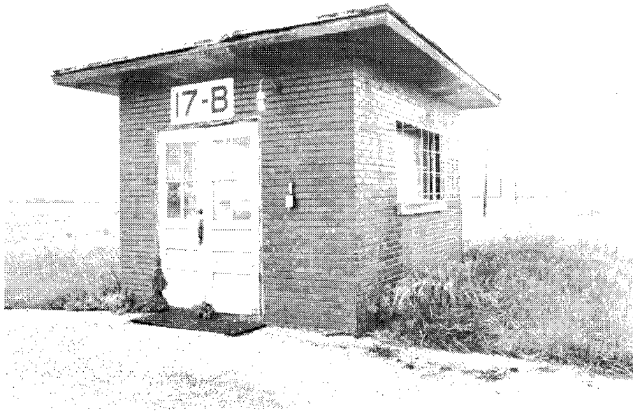
Figure 253. Building 17B: Well Pump Station.
