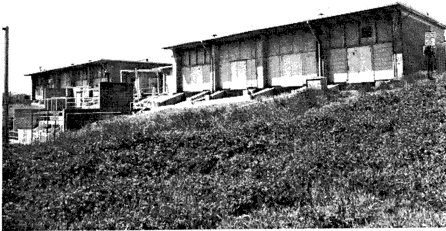
Figure 191. Building 81: Disposal Tanks Building.
