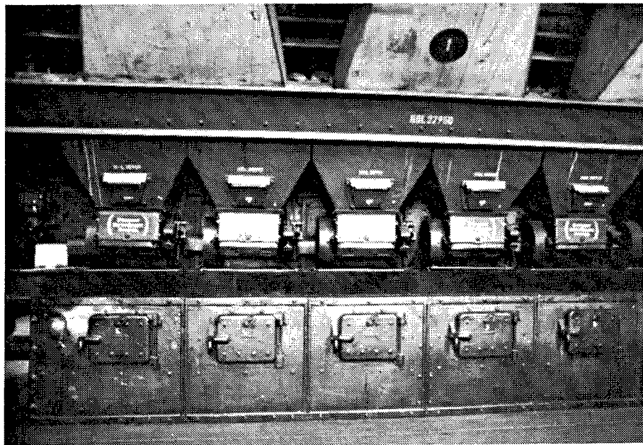
Figure 219. Building 200: Close-up of Detroit RotoGate Stoker No. 1.
