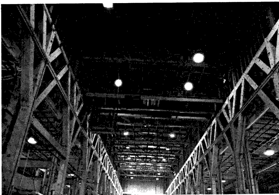
Figure 167. Building 100: View of Rafter Construction and Overhead Bridge Crane with 7.5 ton lift capacity manufactured by Chisholm-Moore Hoist Corp., Tonwanda, NY.
