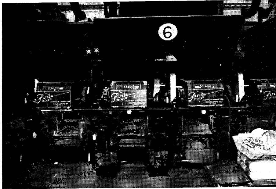
Figure 236. Building A8: Firite Stokers manufactured by the Hoffman Combustion Engineering Co., Detroit, MI.
