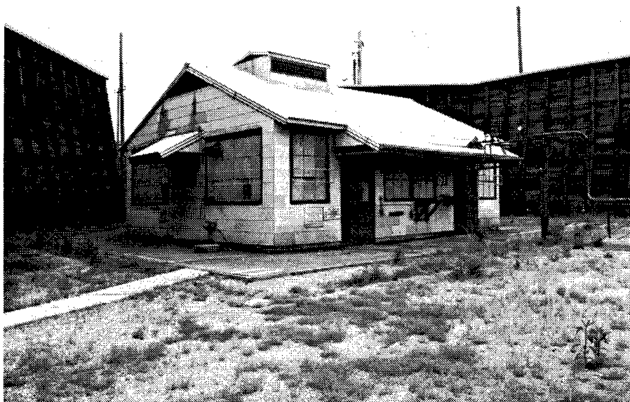
Figure 181. Building O1: Ammunition Quality Control Facility, Explosives Laboratory with double-riveted barricades.
