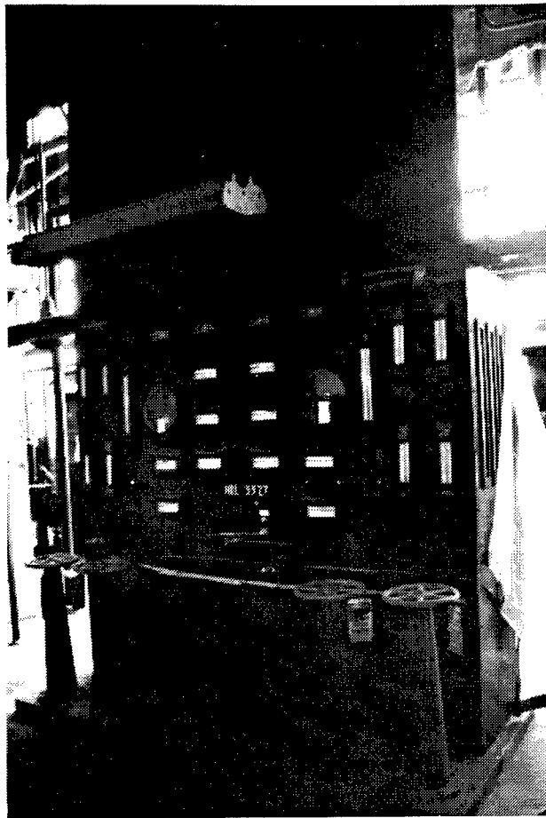
Figure 69. Building A20: Control Panel for Acetic Anhydride Furnaces.
