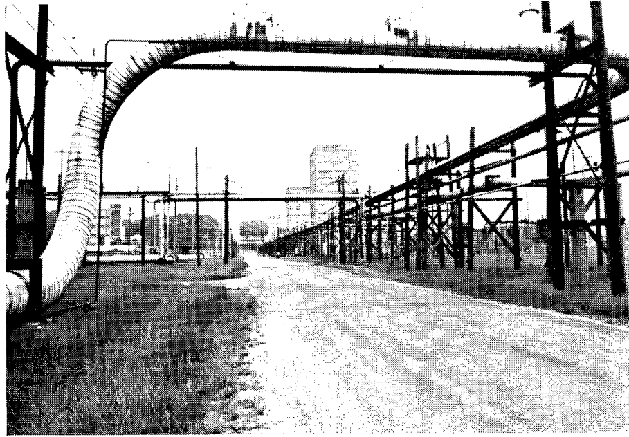
Figure 35. Overhead Acid Pipeline.
