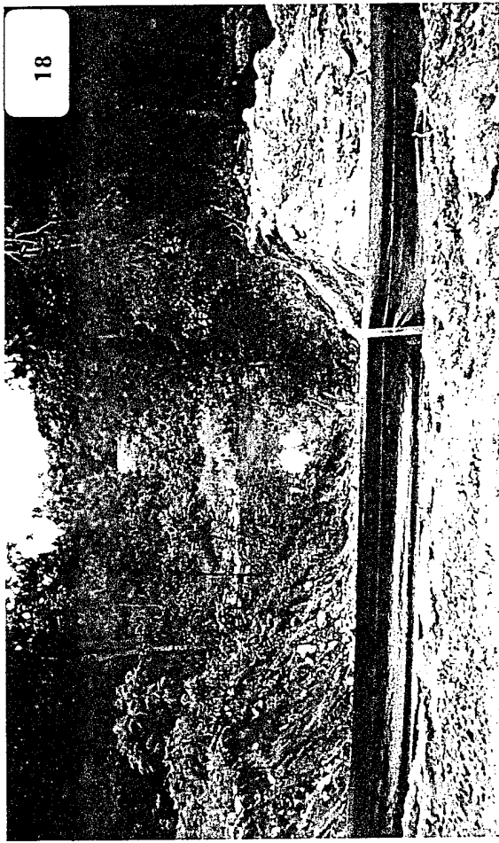
Site 4. Excavation of the gully. Silt fence prevents erosion from the excavations from entering the sinkhole. Photo Date: 7/26/95. Photo Direction: S.
