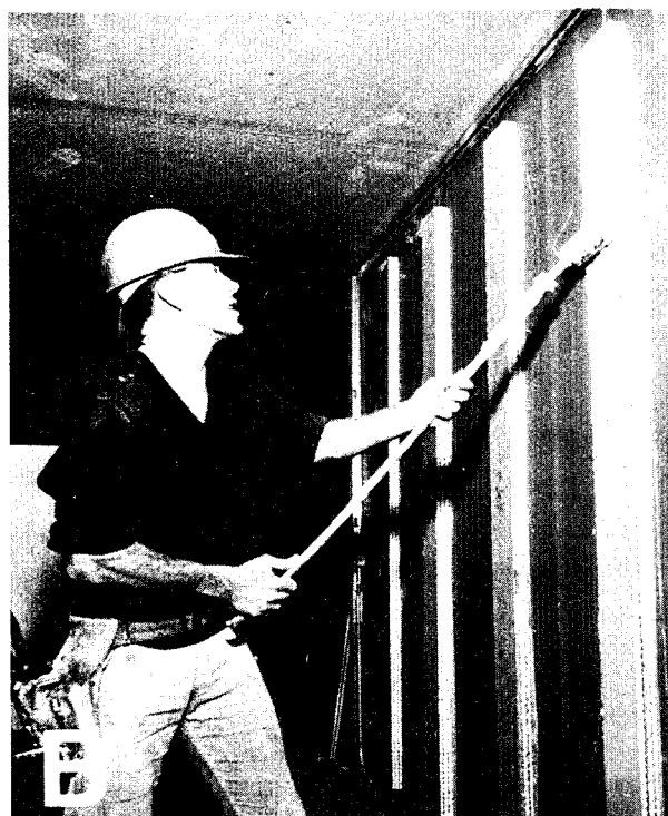
Figure 64.—Simple applicators may be adequate for certain adhesive applications: A, a trowel is used to spread adhesive in preparation for finish flooring; B, a long-handled brush spreads adhesive on furring strips to bond paneling.
