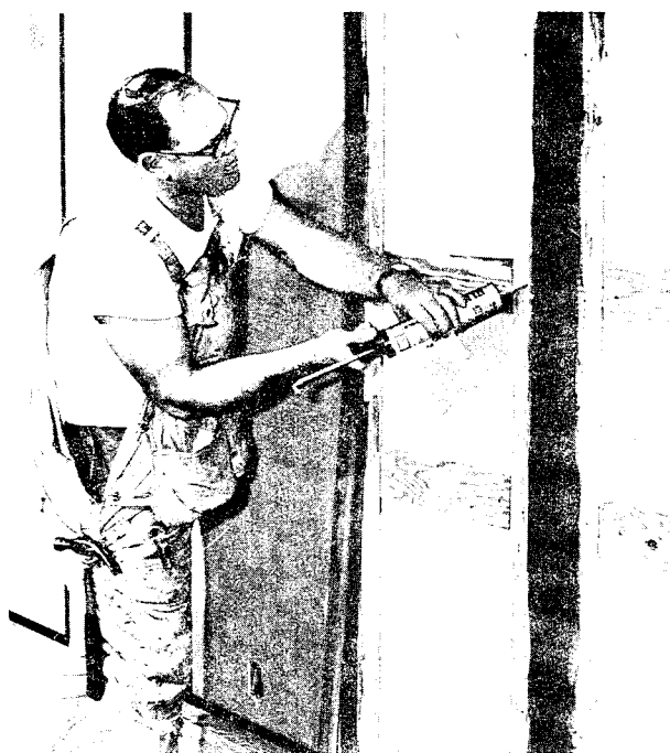
Figure 18.—Application of mastic adhesive to studs for bonding wall panels.
