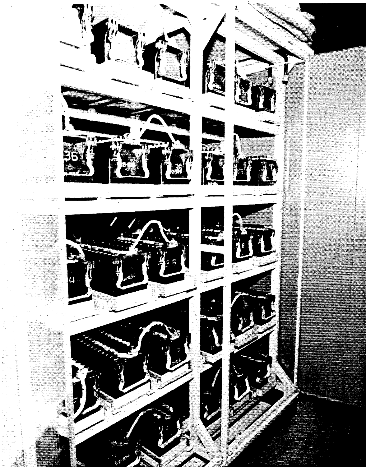
Figure 26 IES Cabinet with the Batteries Installed
