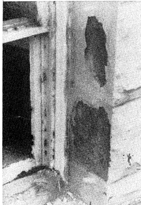
Figure 8. View of wall showing spalling damage to sandstone
