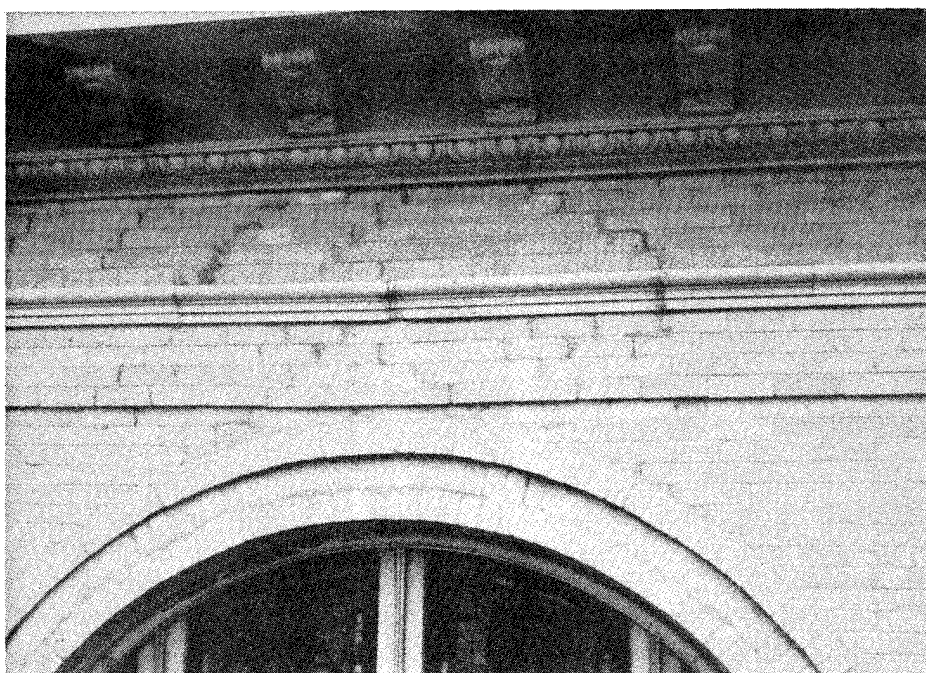
Figure 39. Cracks over arch window in west facade
