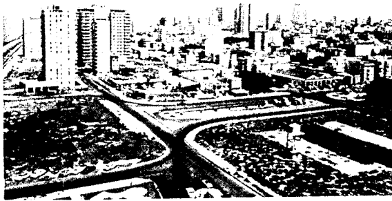
Reinforced concrete and masonry buildings are prevalent in Havana City.
