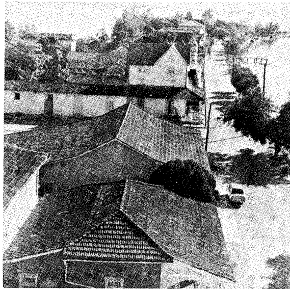
Buildings of stucco-coated brick or masonry are common in the towns of Cuba. Most are single story and have tile floors, and tile or metal roofs.
