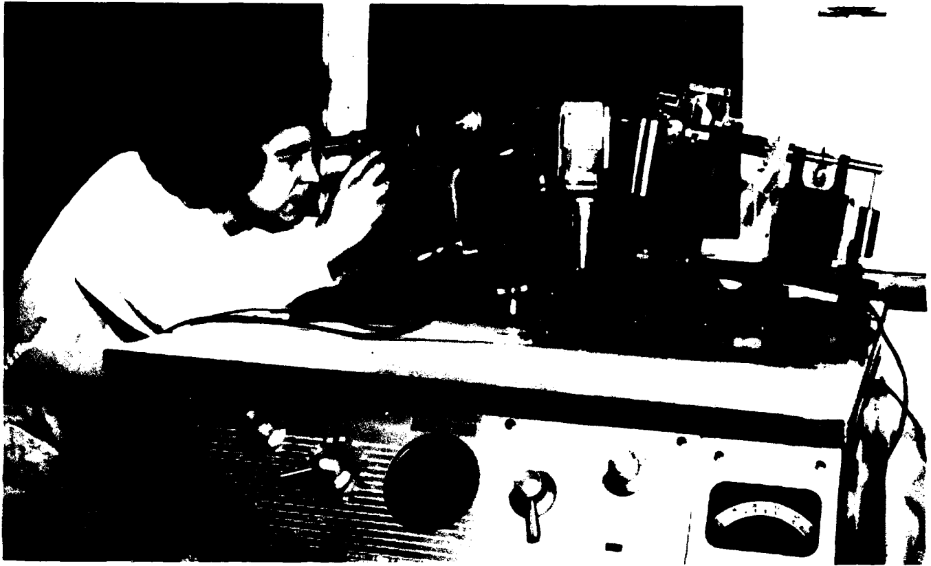
Dr. Karle aligning a crystal on an X-ray camera in the late 1960s.
