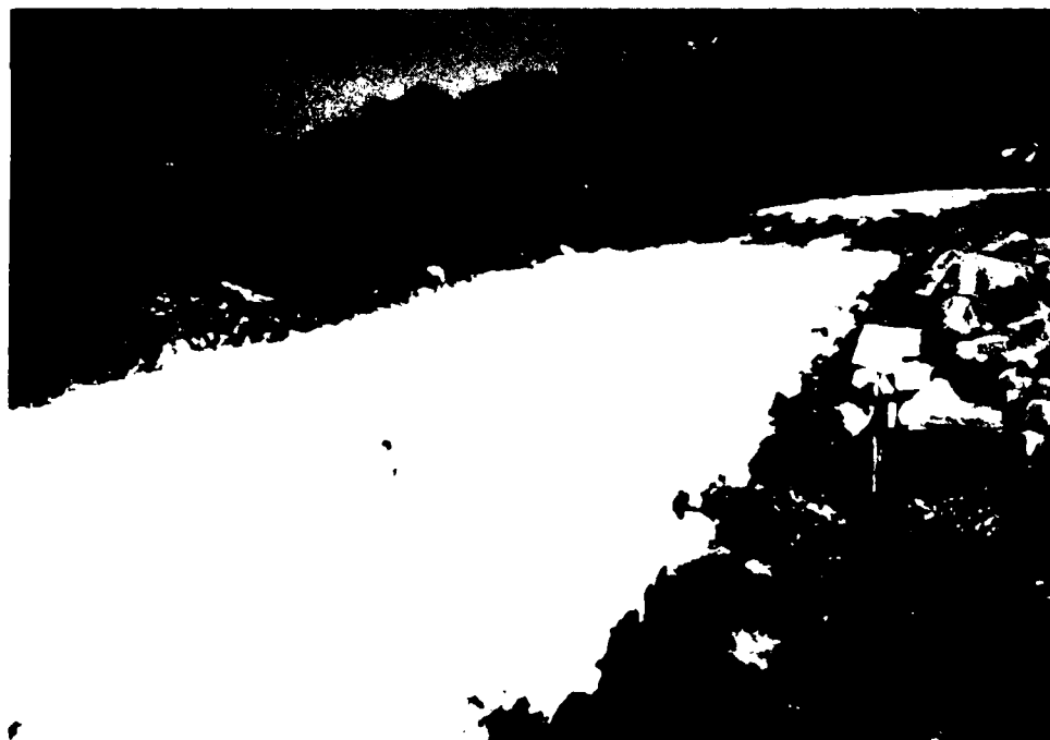
Figure 7. Lime on surface of clay prior to mixing
