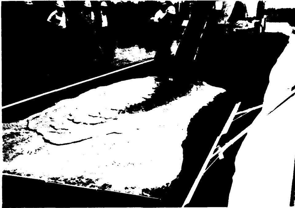
Figure 7. Applying slurry grout to test section
