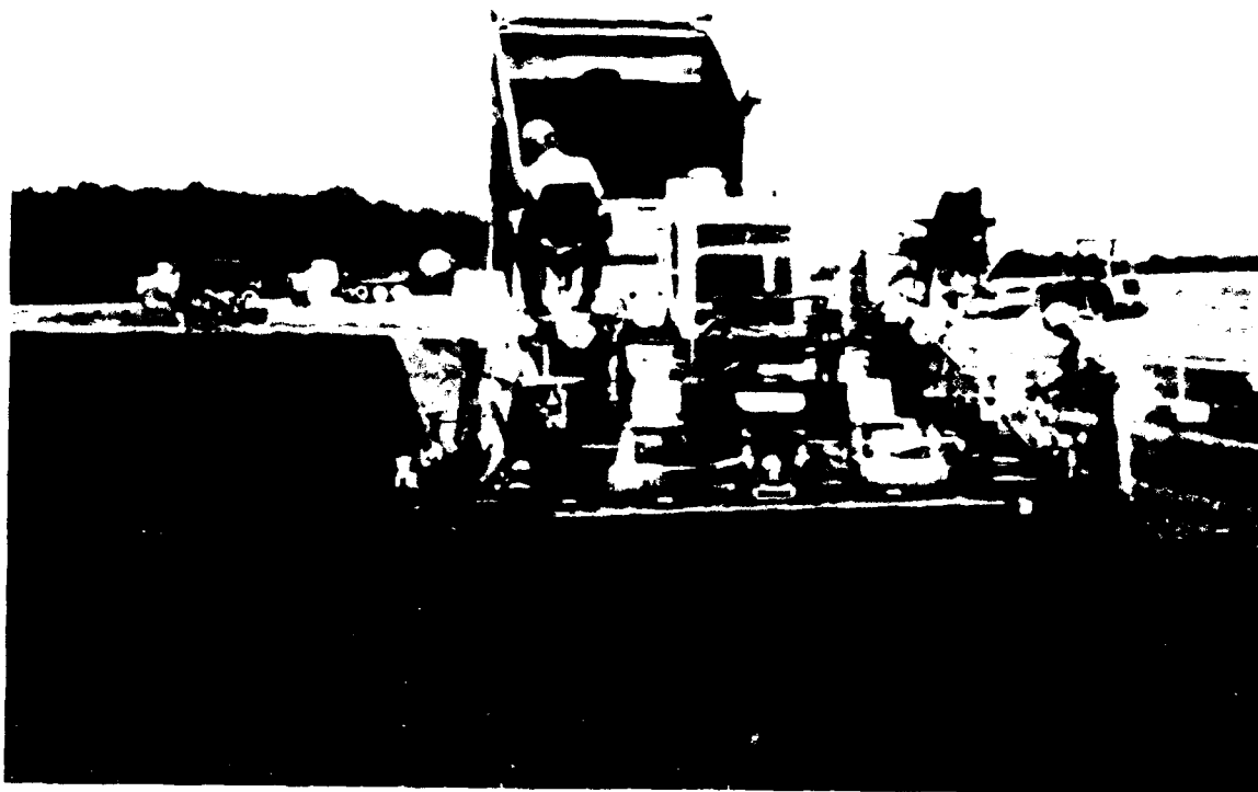
Figure 16. Placement of open-graded asphalt mixture
