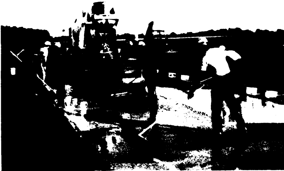
Figure 20. Squeegeeing excess slurry grout over open-graded material
