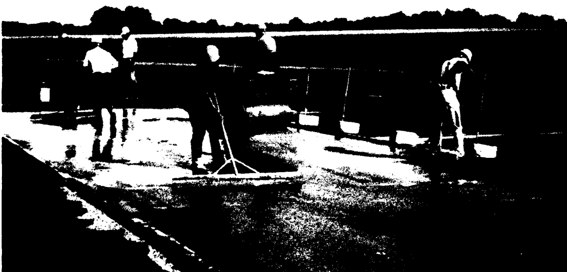
Figure 23. Removing excess slurry grout from surface
