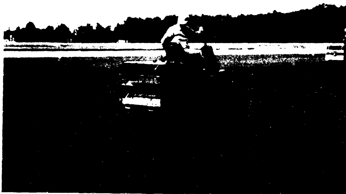
Figure 17. Rolling open-graded material with 3-ton steel wheel rollers
