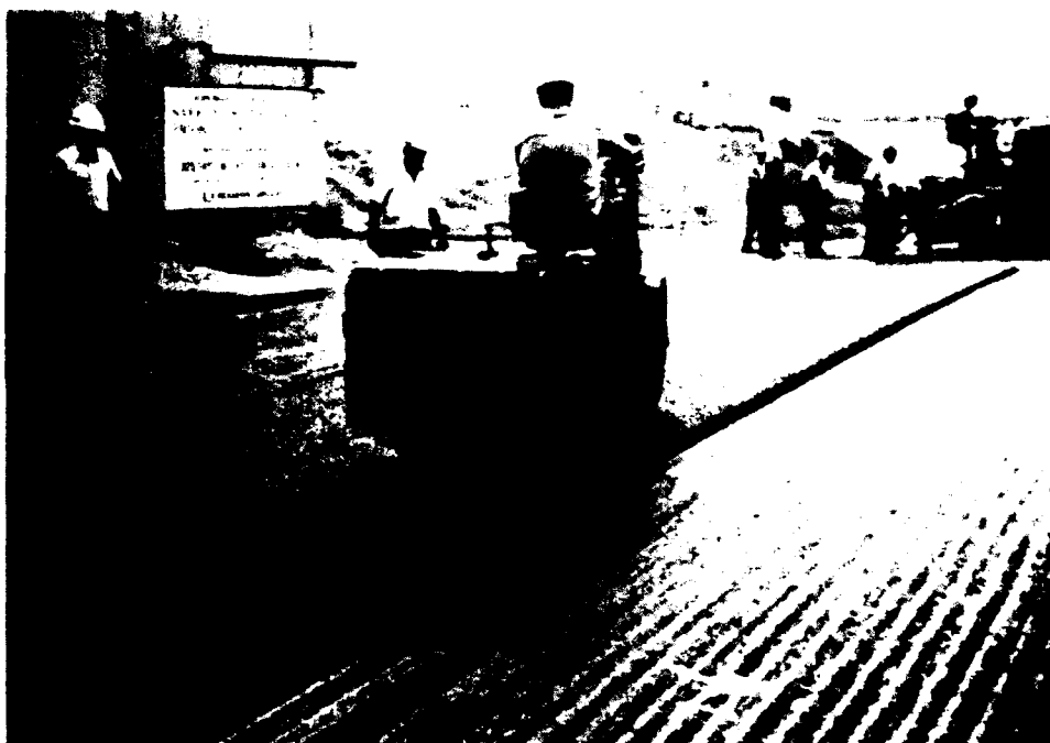
Figure 2. Three-ton steel wheel roller on open-graded material
