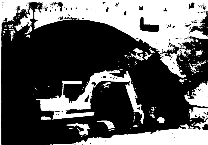
Excavation of transition to springline. Rib C has been set.
