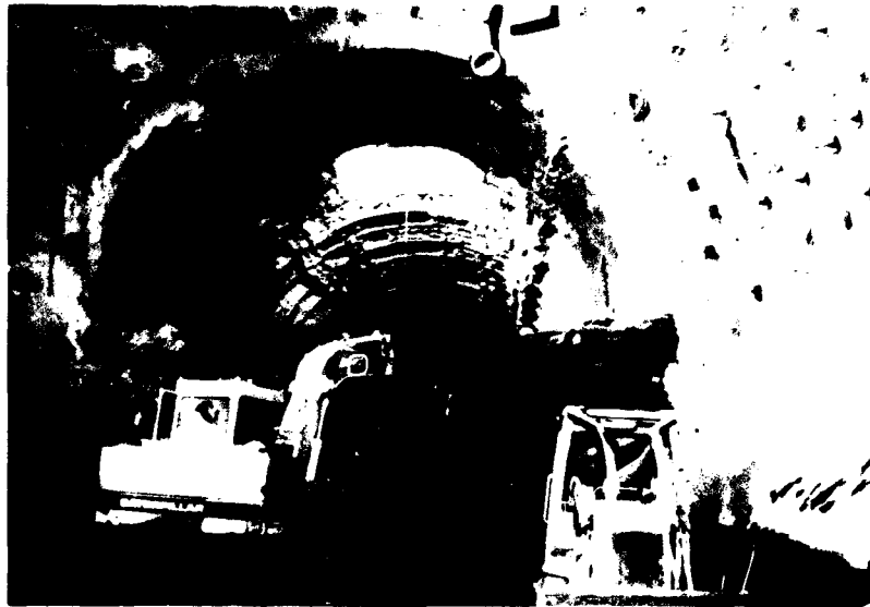
Excavation of lower half of outlet shaft transition.
