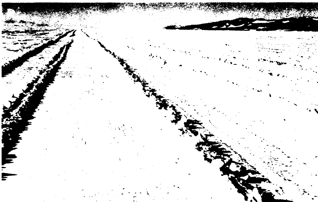
Figure 67. Windrows at the McMurdo Pegasus site. To prepare the snow-on-ice runway, the ice surface was scraped by heavy, long-track bulldozers and the well-mixed snow from the windrows was respread, compacted and graded. (Photo by M. Mellor, January 1990.)
