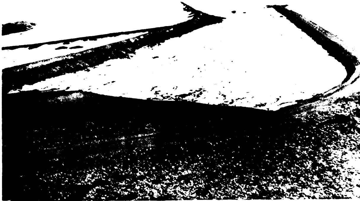
Figure 80. Gravel roads built on glacier ice in Greenland. The road to the right is newly built. The one to the left has deteriorated due to ablation of the adjacent bare ice. The mean annual temperature here is -11^{\circ}\text{C} , and the thaw index is 270–360 ^{\circ}\text{C} degree-days, causing the ice to suffer net ablation of about 8 ft/yr (2.4 m/yr). The optimum depth of gravel fill was 3 ft (0.9 m), with 2.5 ft (0.76 m) of coarse material and 0.5 ft (0.15 m) of fine gravel capping. (U.S. Army photo by SP5 W.J. Davis, 1961.)
