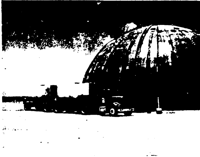
Figure 3.3. ANFO being pumped into hemisphere during filling operation.
