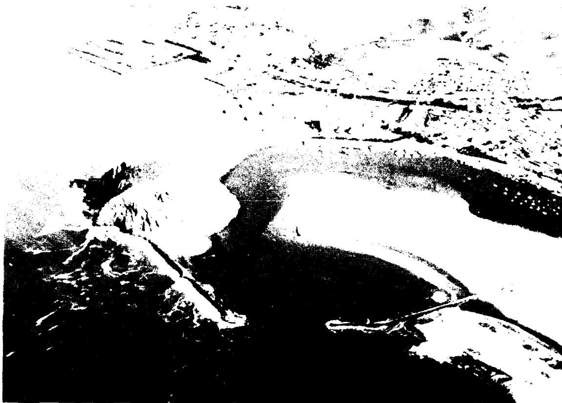
Figure 3. Aerial view of Morro Bay entrance
