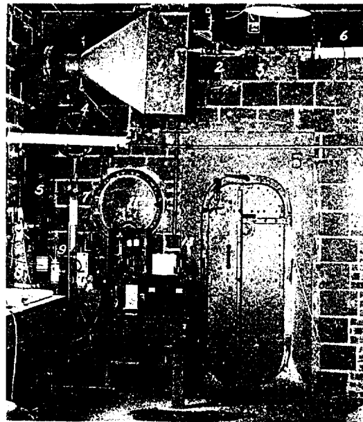
FIGURE 3-4 (A) Naval Research Laboratory (NRL) gas chamber. interior dimensions of this chamber were 10 ft. by 15 ft., with a 12 ft. high ceiling. The chamber was designed to fit ten men and allow room for moderate exercise. (B) Photograph of the inside of a similar gas chamber used at Edgewood Arsenal for World War II chamber tests (the numbers refer to specific equipment). SOURCE: Taylor et al., 1943. Photographs provided by Naval Research Laboratory (A) and U.S. Army Chemical and Biological Defense Agency (B).
