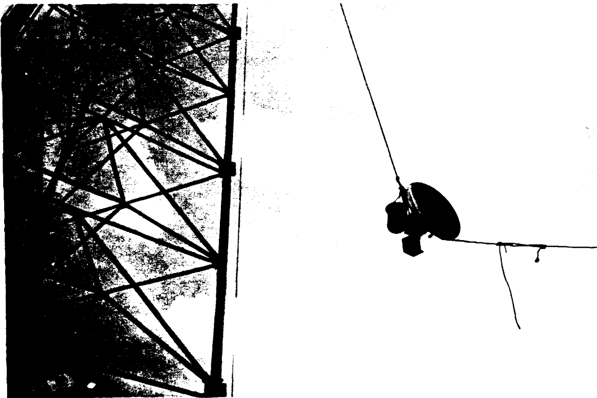
Figure 5. MTS being hoisted to the 170-foot-high tower.
