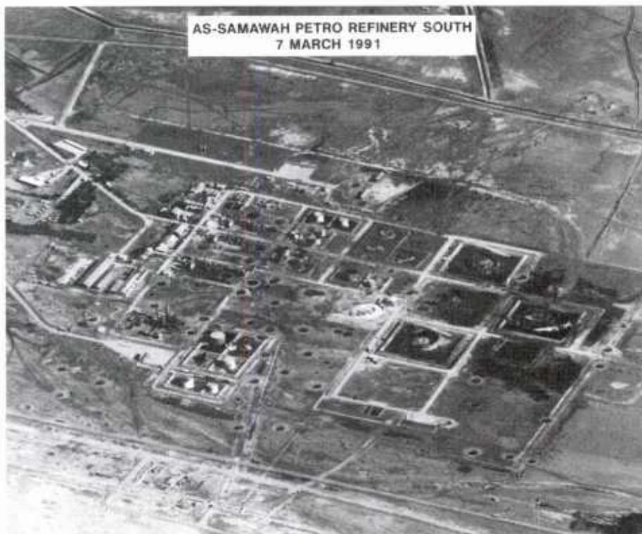
Figure VI-23 As-Samawah Petroleum Refinery (Post-Strike).
