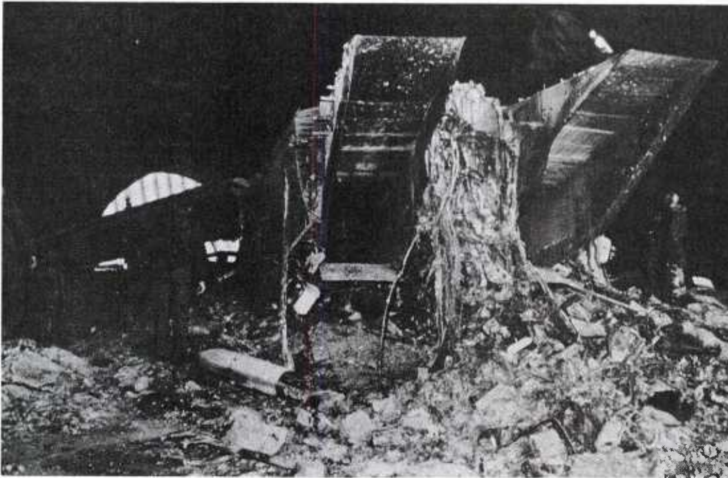
Figure VI-8 Saddam Hussein Tried to Protect His Air Force in Hardened Aircraft Shelters. Penetrating Bombs Denied This Sanctuary.
