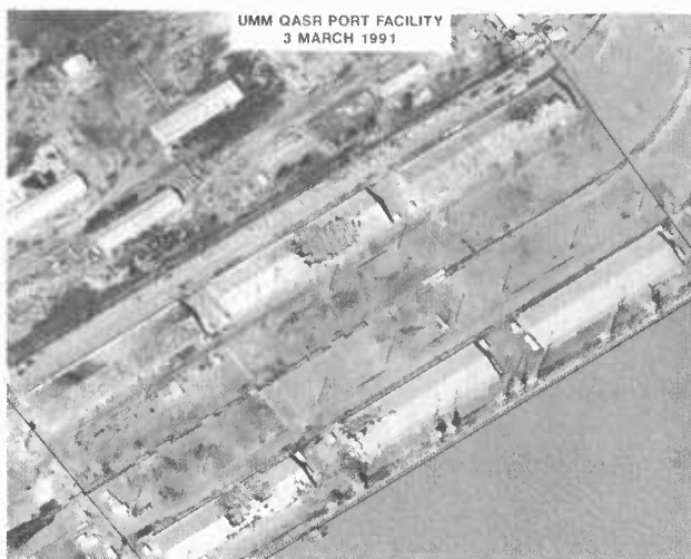
Figure VI-22 Coalition Air Strikes Inflicted Serious Damage to the Umm Qasr Port Facility.
