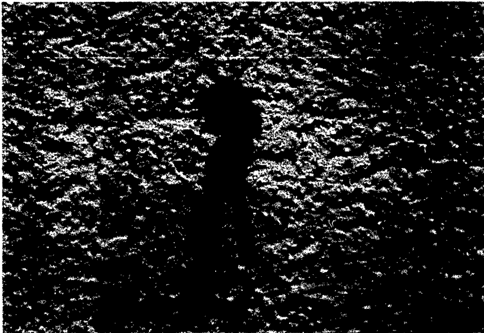
Figure 80. Stains due to finish coat impurities.
