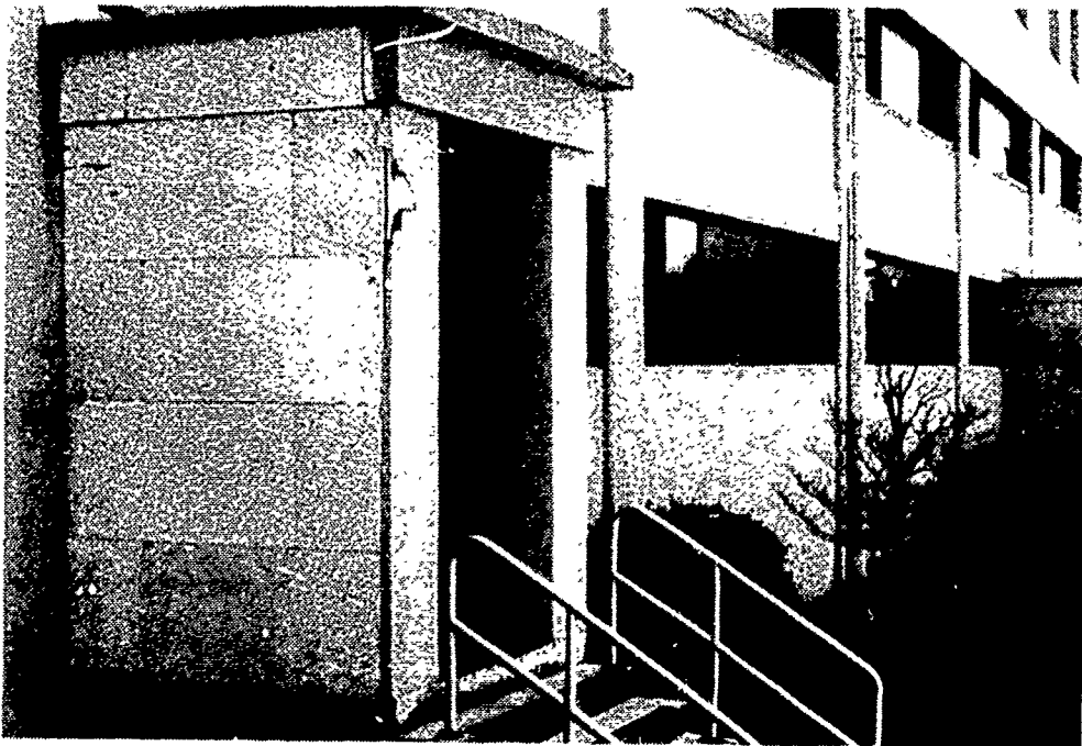
Figure 34. Ultraviolet EPS board damage.
