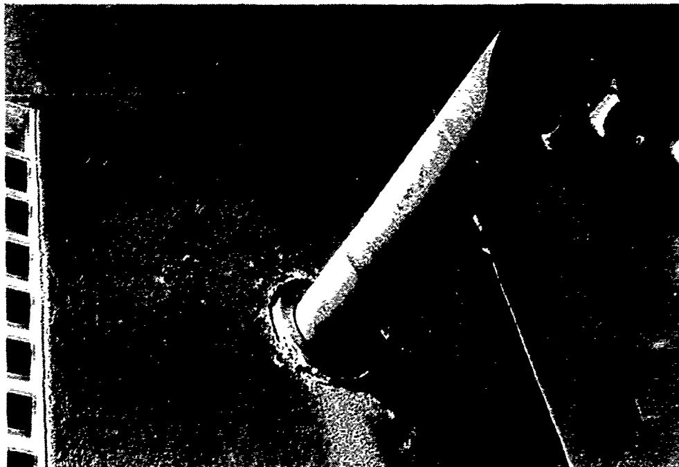
Figure 52. Inadequate closure at pipe.
