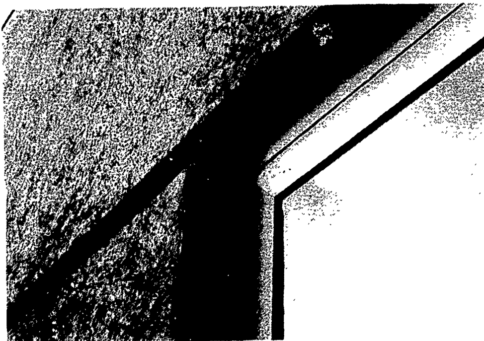
Figure 12. Cracking in "U" groove articulation.
