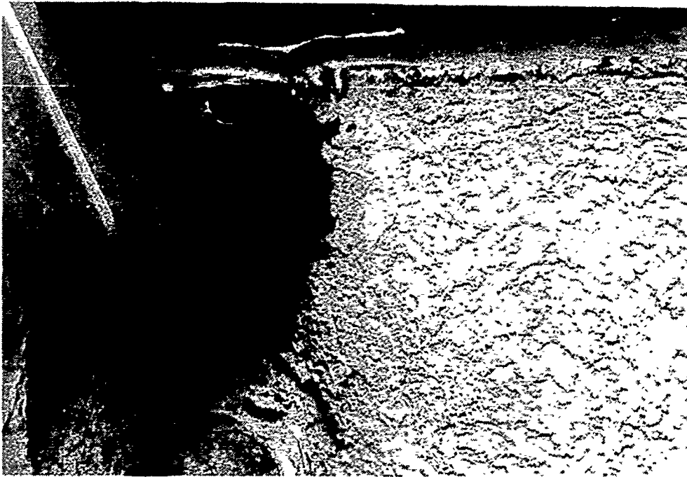
Figure 50. Inadequate closure at pipe.
