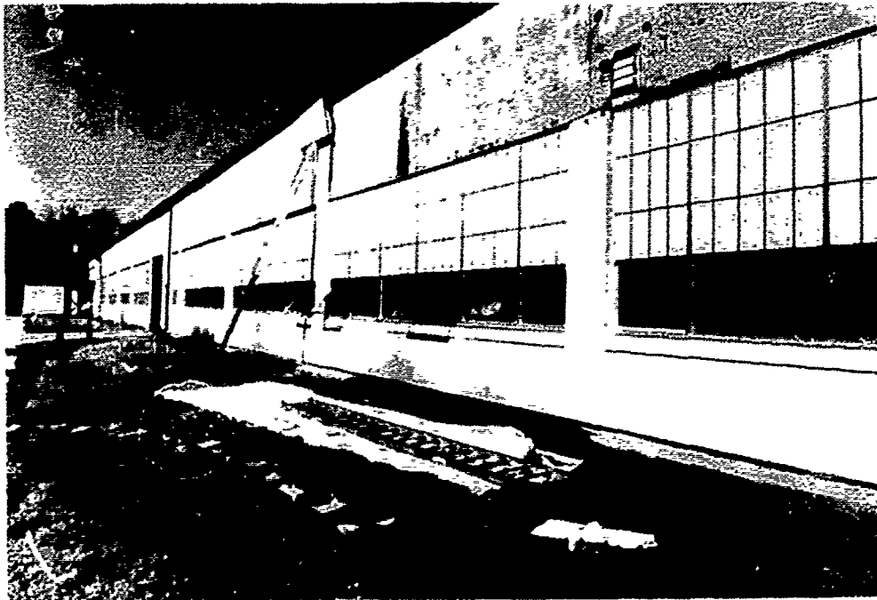
Figure 68. Catastrophic system detachment.
