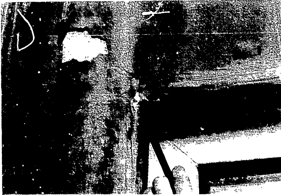
Figure 31. Spalling of base coat due to improper application.
