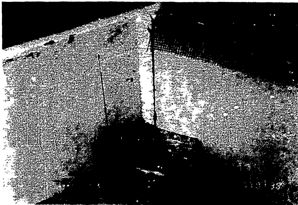
Figure 61. Good EIFS termination — incorrect backwrap.
