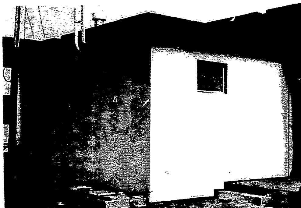
Figure 75. Stains due to laundry room exhaust.
