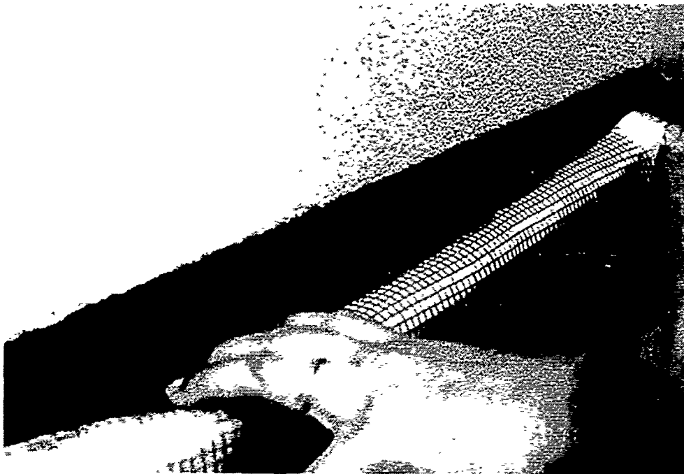
Figure 66. Insufficient adhesive attachment.
