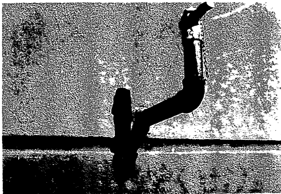
Figure 49. Inadequate closure at pipe.
