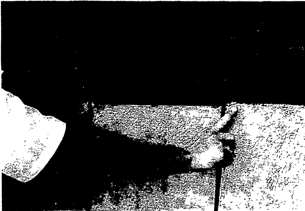
Figure 21. Premature control joint termination.
