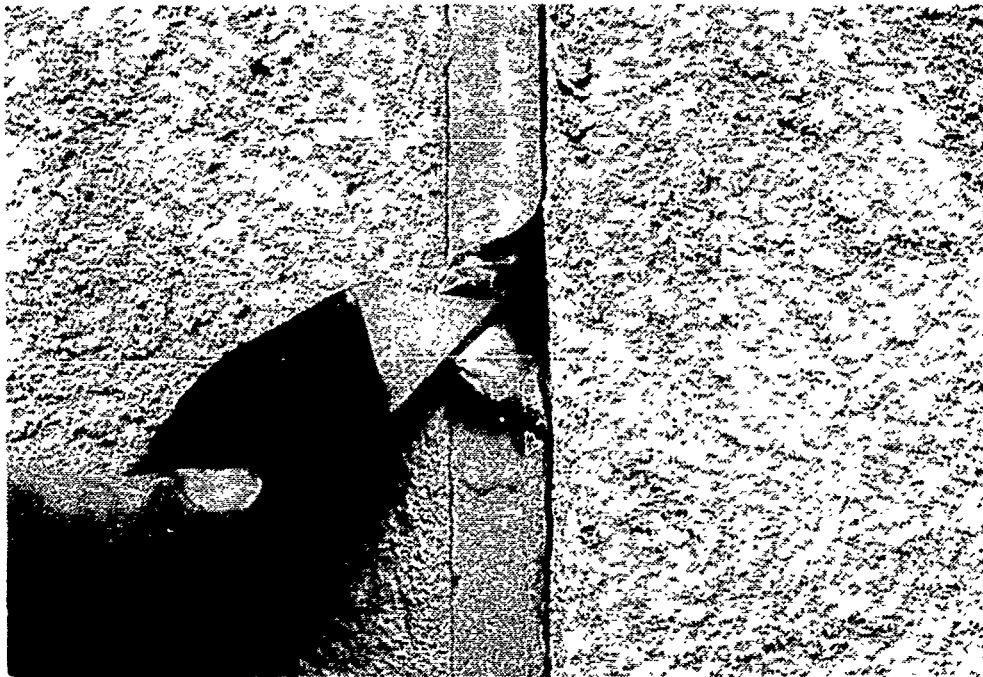
Figure 64. Cohesive and adhesive sealant failure.
