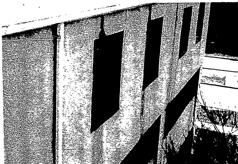
Figure 74. Stains due to leaks in gutter.
