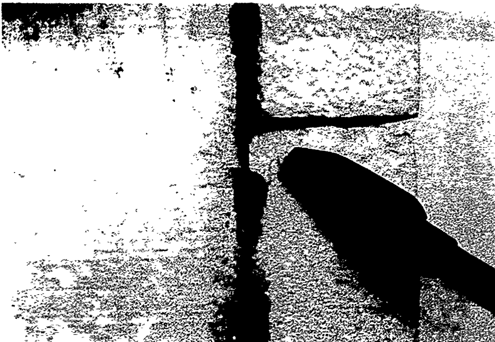
Figure 5. Adhesive between EPS boards - improper.
