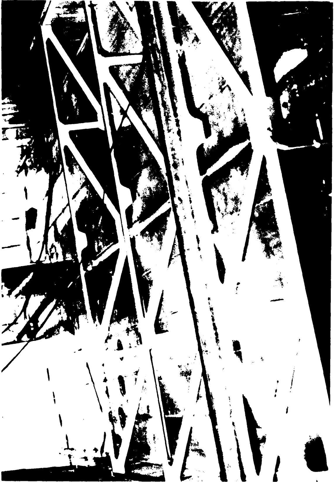
Figure 6. Installation of Internal Trusses
