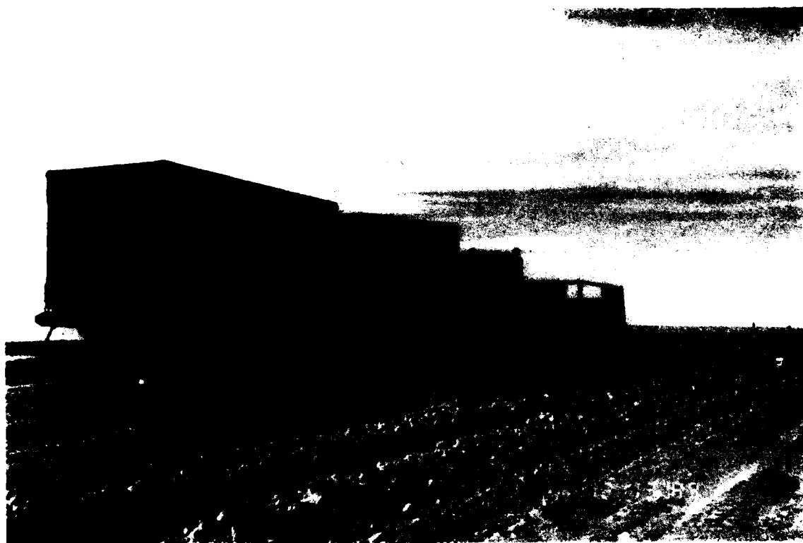
Figure 25. Portable airfield buildings mounted on Otaco sleds.
