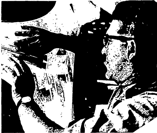
Figure 47. Sealing of joint space between spherical pentagons prior to bonding.
