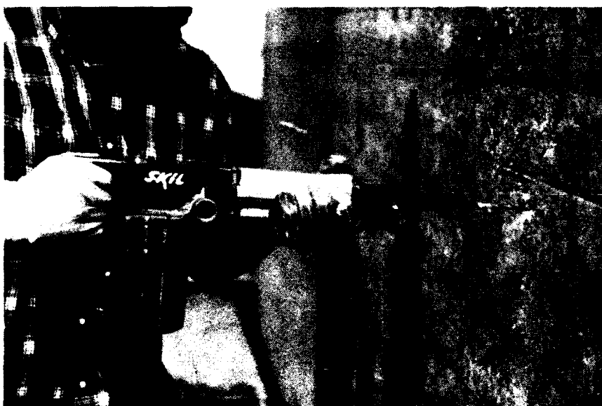
Figure 19. Predrilling of port holes
