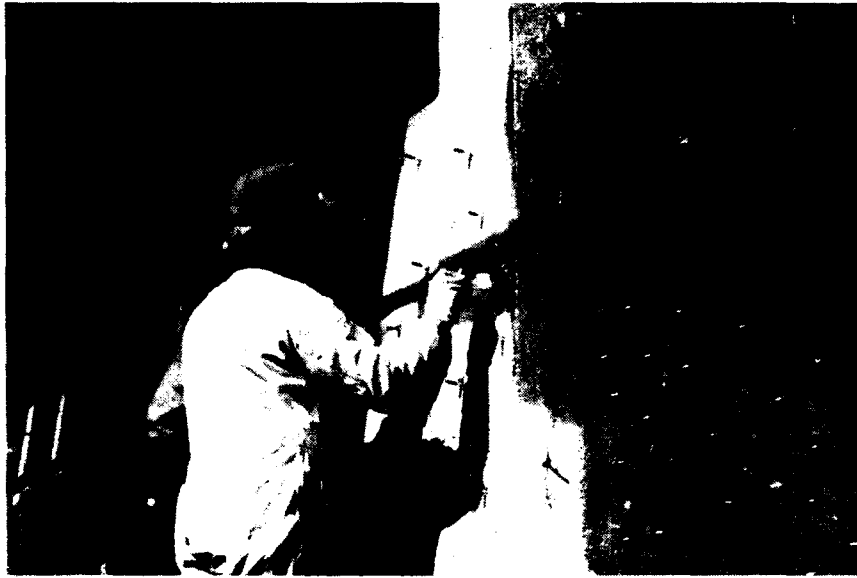
Figure 24. Application of epoxy seal coat
