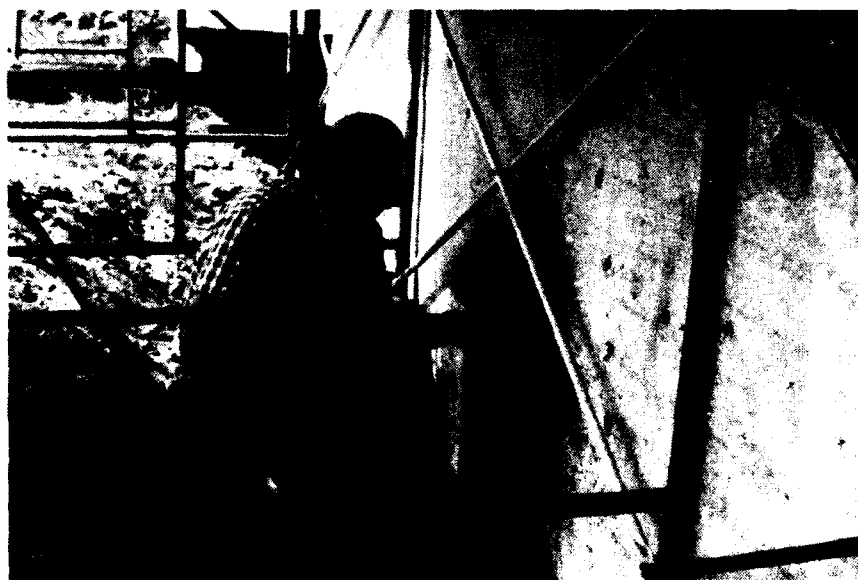
Figure 17. Drilling of port holes using the CP-9RR rock drill
