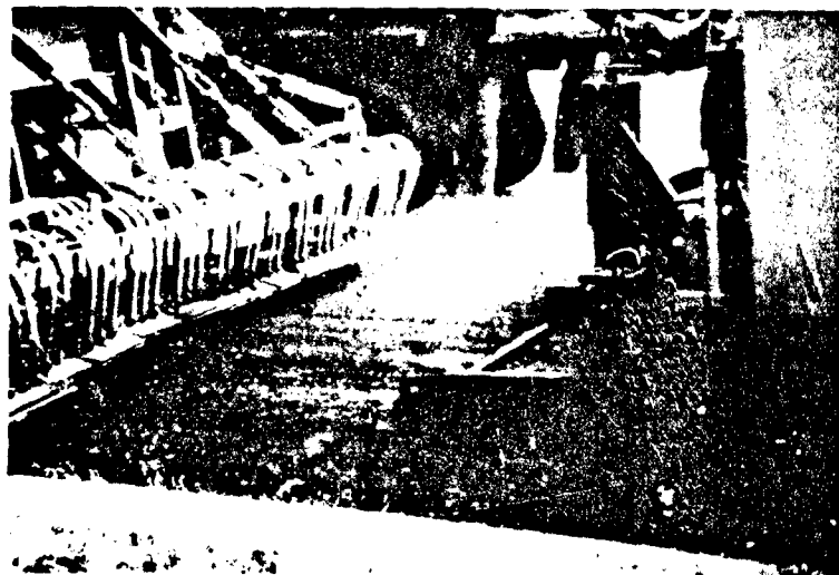
Photo 32. Spray bar for applying rejuvenator
