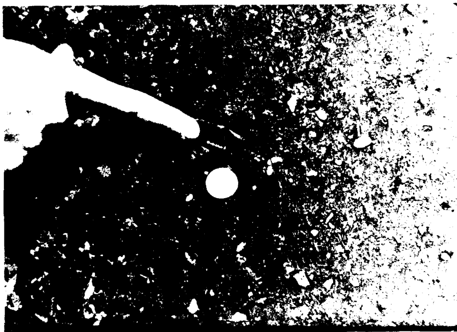
Figure A5. Low-severity bleeding.
