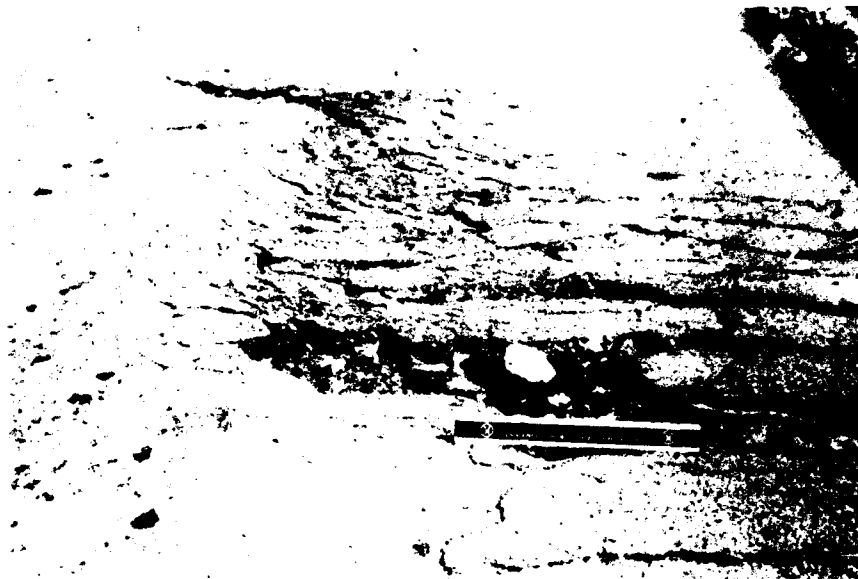
Figure A50. High-severity slippage cracking.
