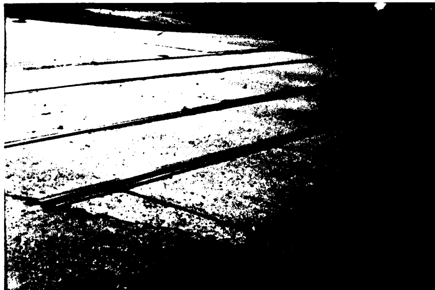
Figure A94. Low-severity railroad crossing.
