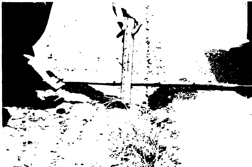
Figure A27. Medium-severity lane/shoulder drop-off.
