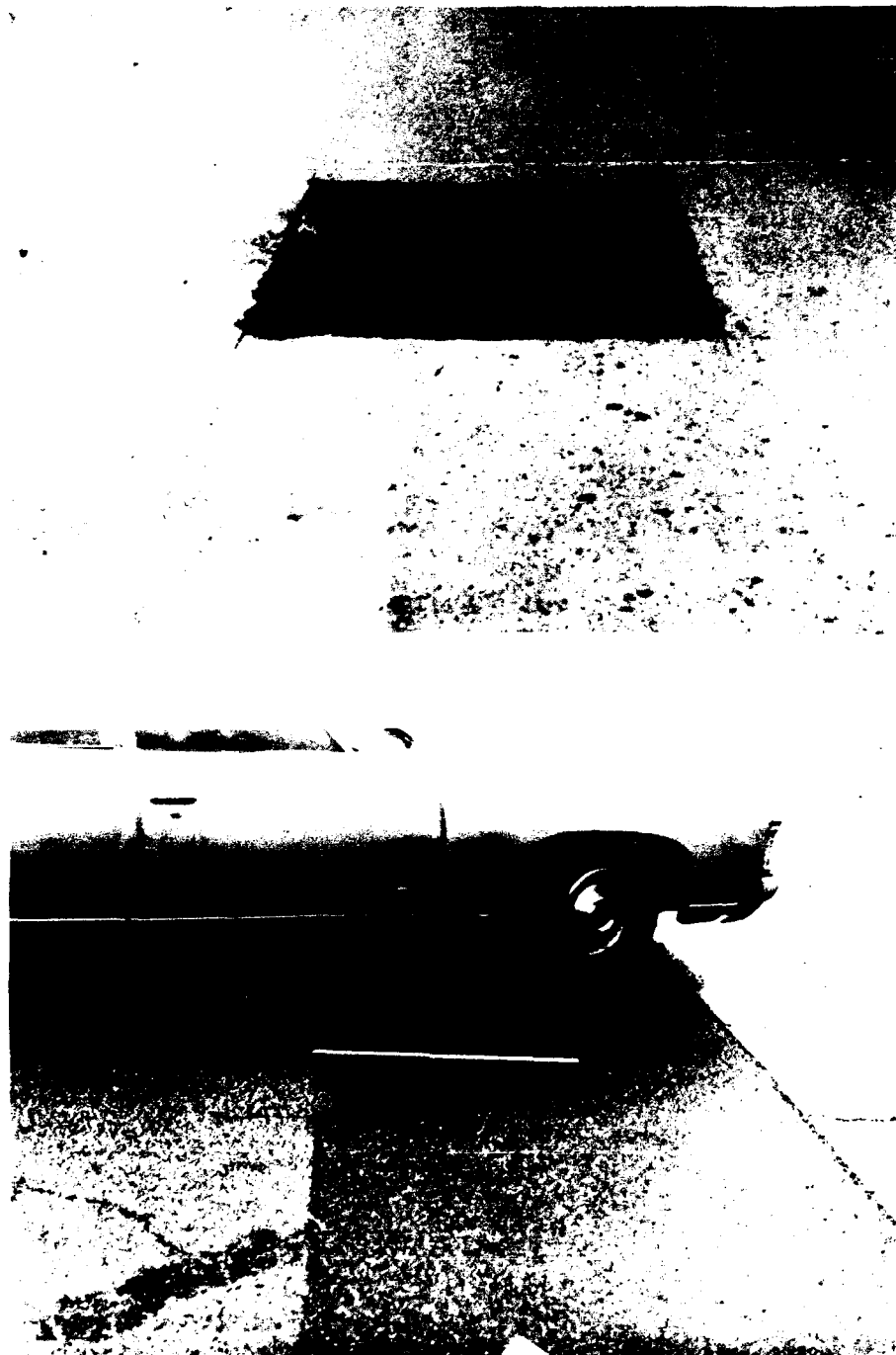
Figure A32. Examples of low-severity patching and utility cut patching.
