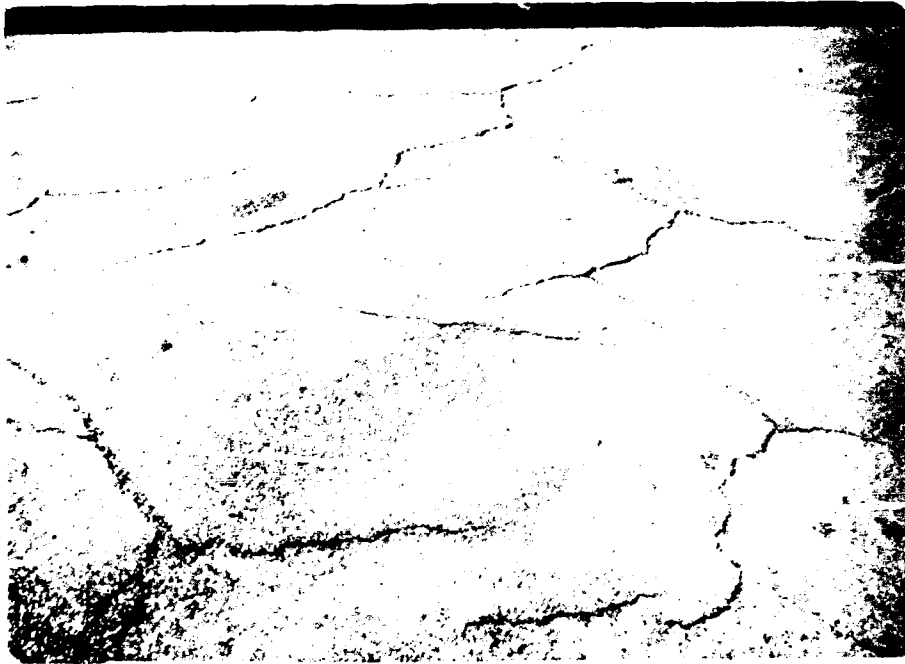
Figure A8. Low-severity block cracking.
