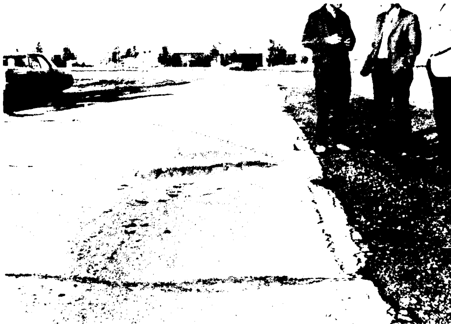
Figure A11. Low-severity bumps and sags.
