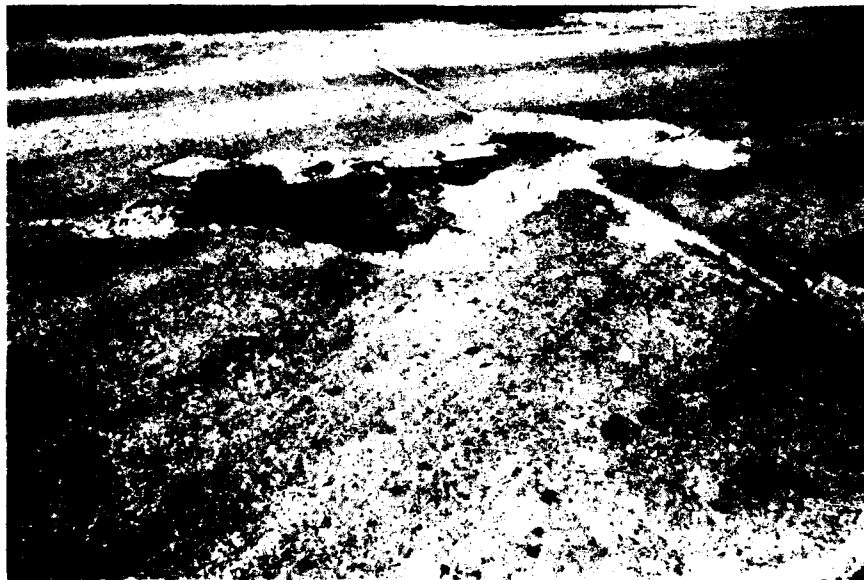
Figure A99. Examples of high-severity scaling/map cracking/crazing.
