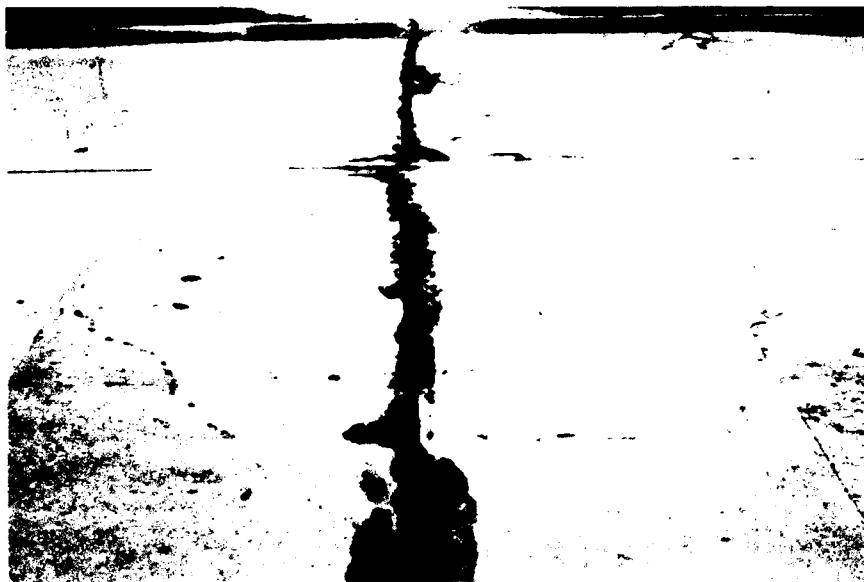
Figure A72. Low-severity joint seal damage.
