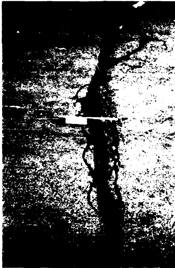
Figure A25. High severity joint reflection cracking.
