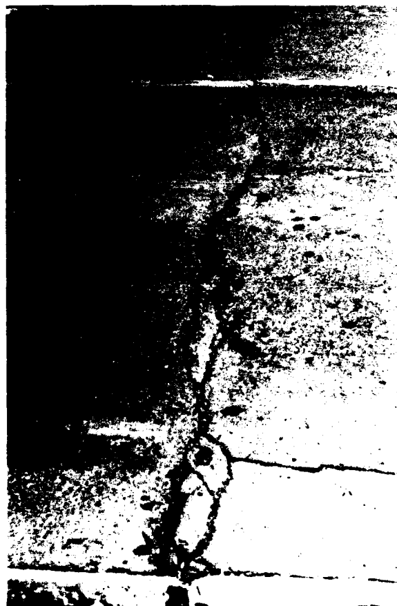
Figure A24. Medium-severity joint reflection cracking.
