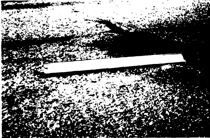
Figure A11. Low-severity bumps and sags.
