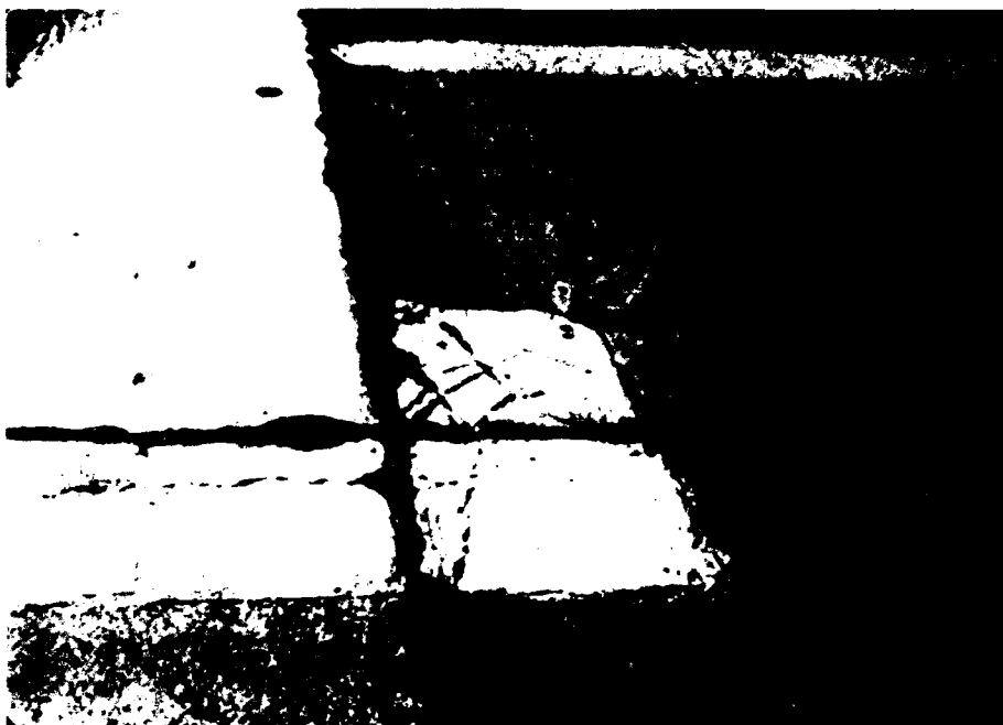
Figure A86. Medium-severity patching (small).
