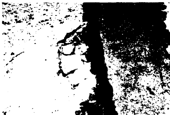
Figure A56. Low-severity blowup/buckling.
