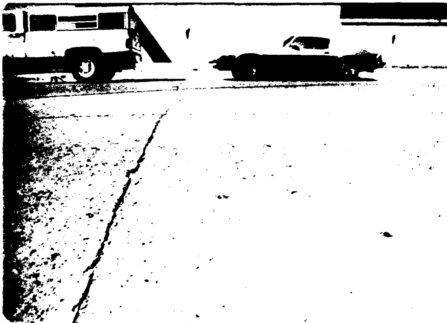
Figure A104. Low-severity joint spalling.
