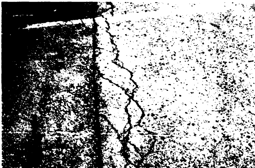
Figure A21. Medium-severity edge cracking.
