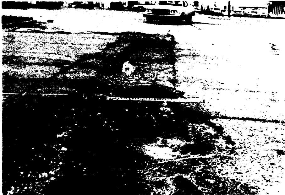
Figure A34. High-severity utility cut patching.
