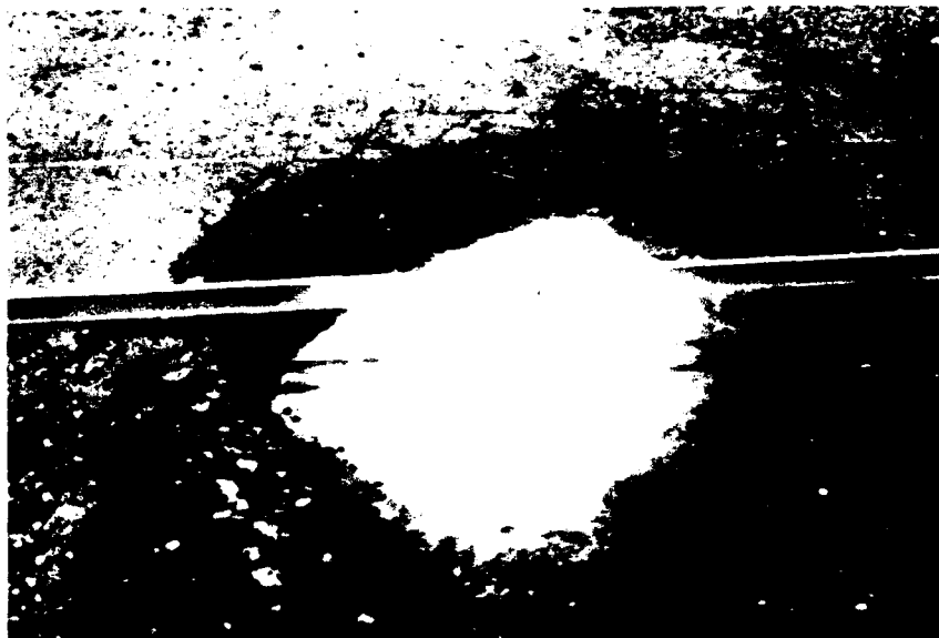
Figure A38. High-severity potholes.
