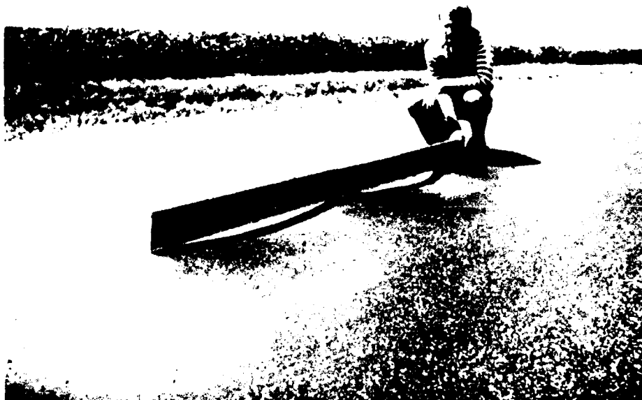
Figure A16. High-severity corrugation.
