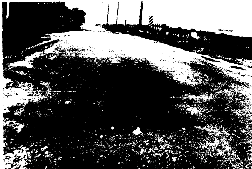
Figure A46. Medium-severity shoving approaching high severity.
