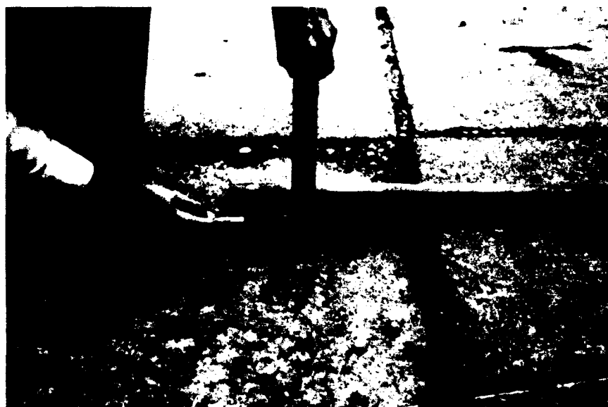
Figure A71. High-severity faulting.
