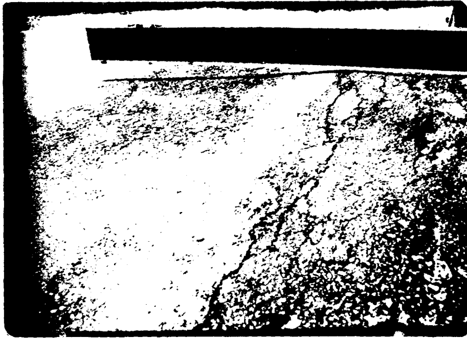
Figure A13. High-severity bumps and sags.
