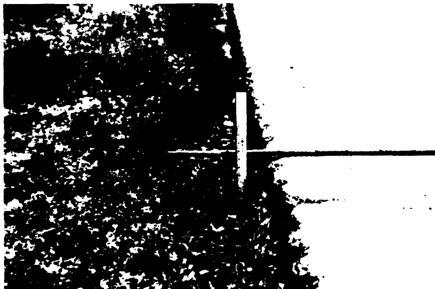
Figure A28. Examples of high-severity lane/shoulder drop-off.
