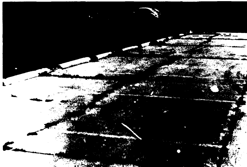
Figure A63. Medium-severity divided slab.
