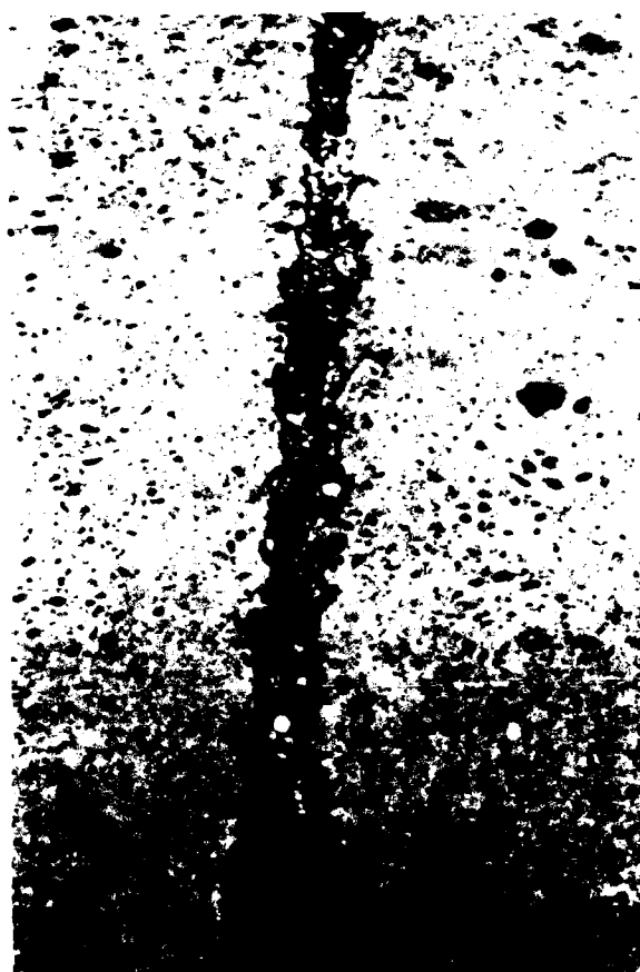
Figure A74. Examples of high-severity joint seal damage.
