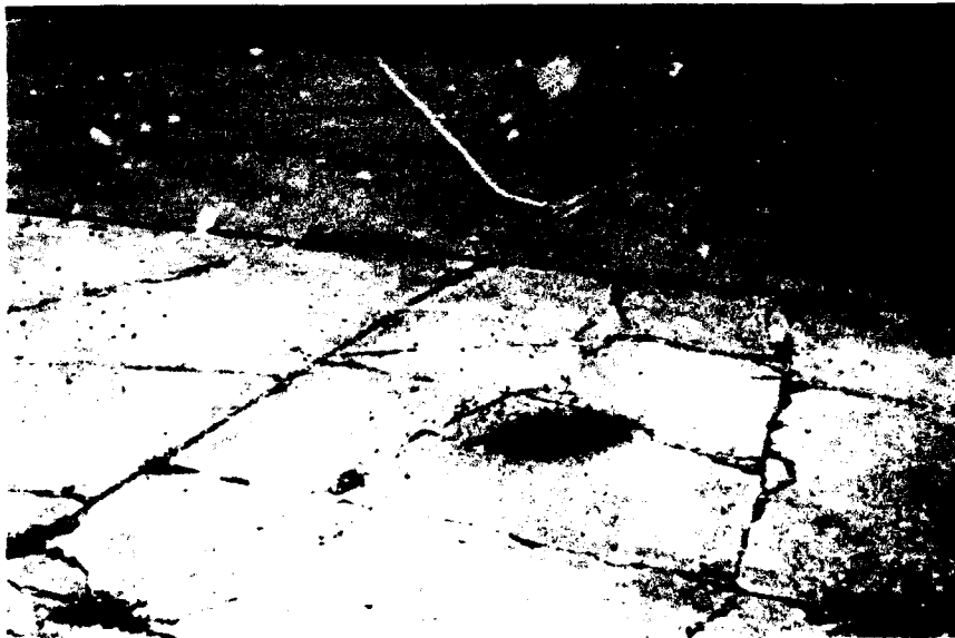
Figure A65. More examples of high-severity divided slabs.
