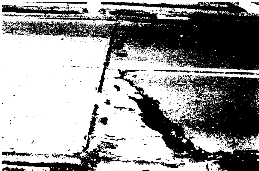
Figure A91. Low-severity punchout.
