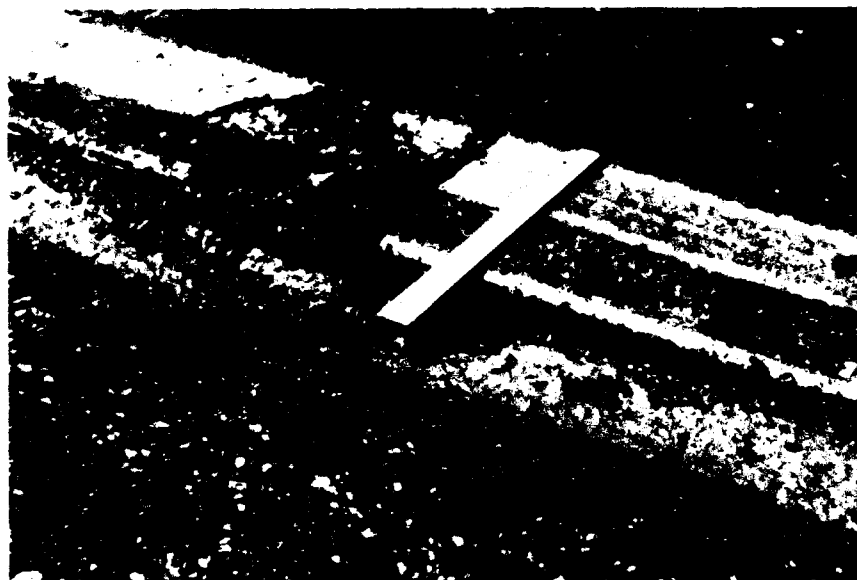
Figure A75. Low-severity lane/shoulder drop-off.
