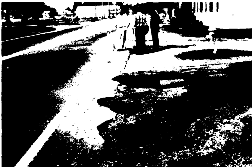
Figure A22. Examples of high-severity edge cracking.
