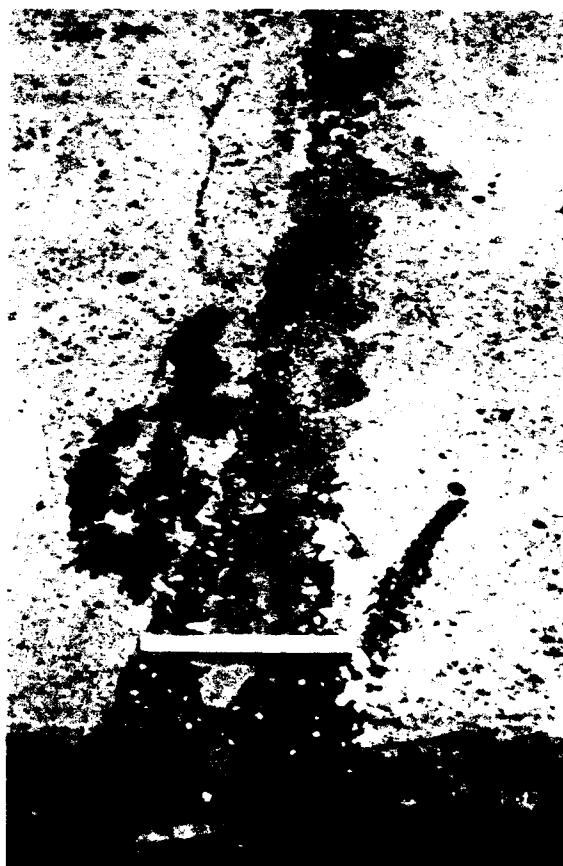
Figure A80. Examples of high-severity linear cracking in nonreinforced concrete slab.
