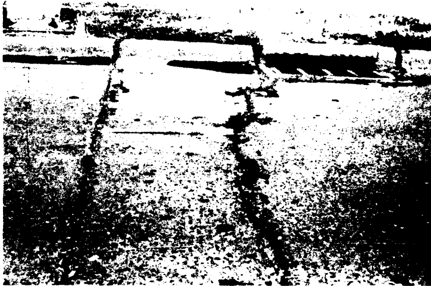
Figure A91. Low-severity punchout.
