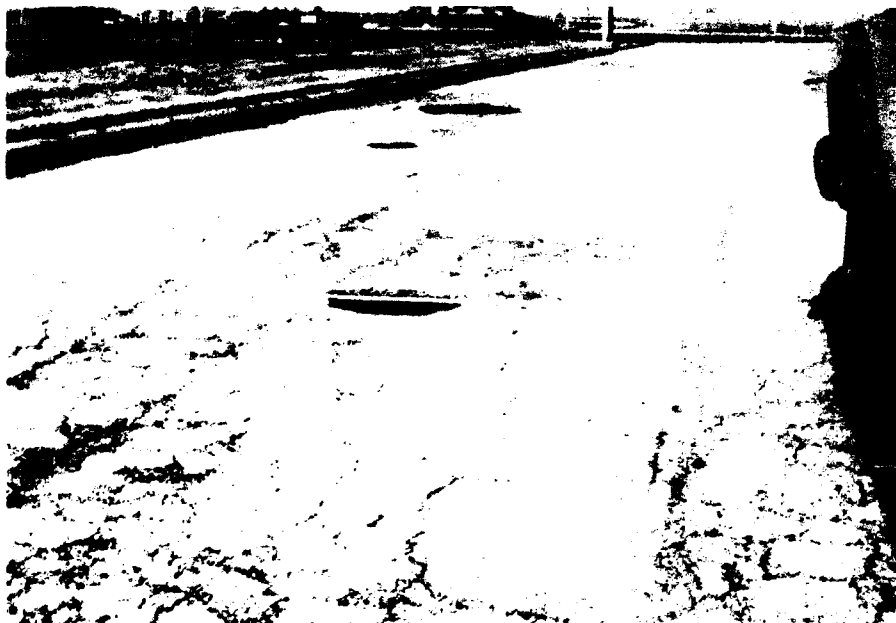
Figure A37. Medium-severity pothole.
