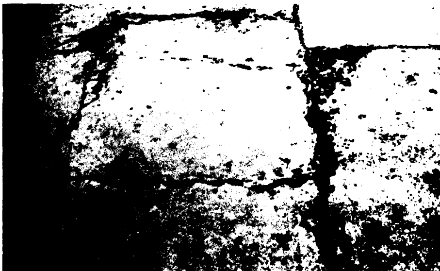
Figure A84. High-severity patching (large).
