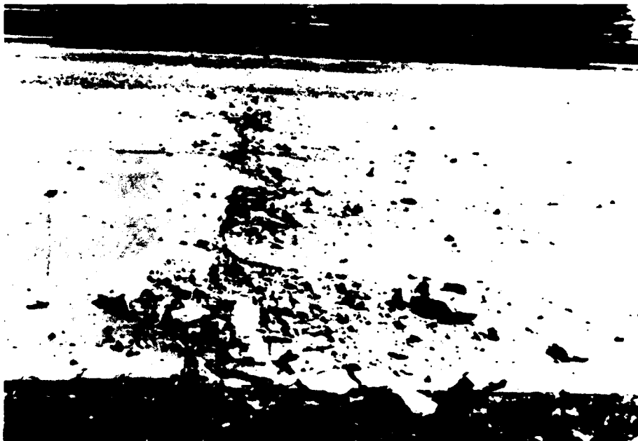
Figure A57. Examples of medium-severity blowup/buckling.
