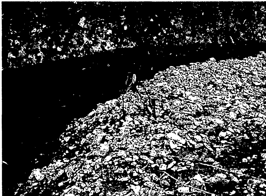
Figure C12. Channel erosion. Note exposed bank materials on outside curve with material accumulation on inside curve (foreground).
