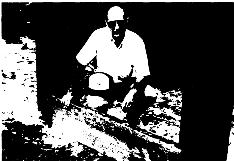
Figure 5. Outlet structure showing method of installing weir boards
